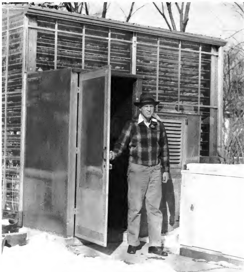
New all-plastic and aluminum time-lapse greenhouse. Double vestibule doors provide both light trap and wind break so that pictures are not spoiled if automatic timer should operate while door is open.
