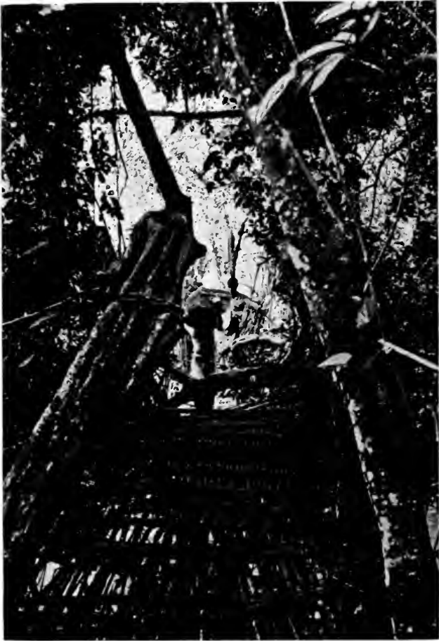
BRIDGE OF CREEPERS OVER LUFUKO RIVER
