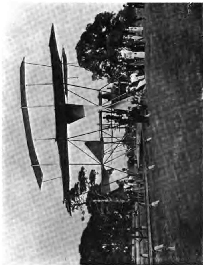
THE FLYING MACHINE WITH THE SIDE WINGS REMOVED
