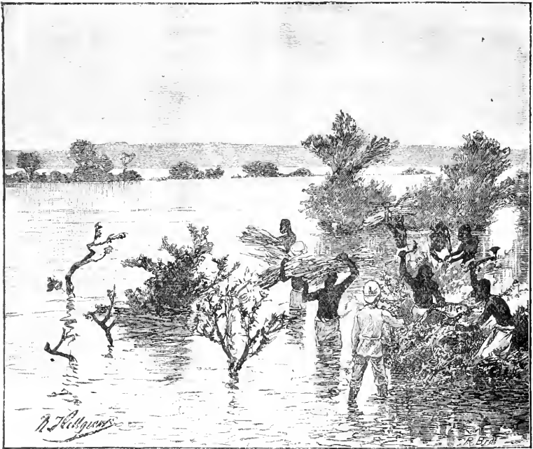
BUILDING OF A BRIDGE
