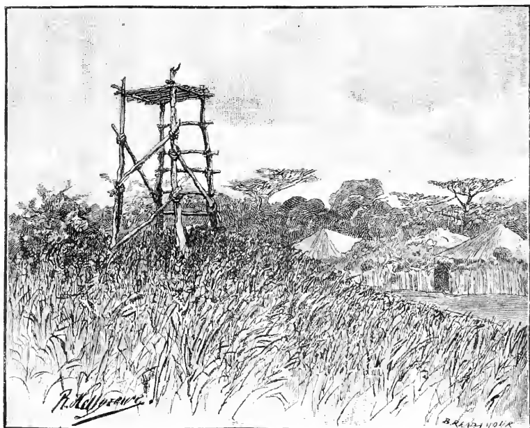
WATCH-TOWER NEAR BISSISSI
