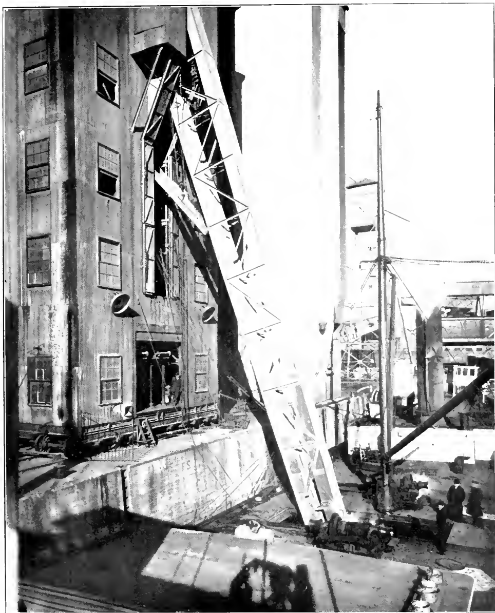
Unloading S.S. "Midland Queen" into No. 1 Harbour Commissioners Elevator, Montreal, Canada.
