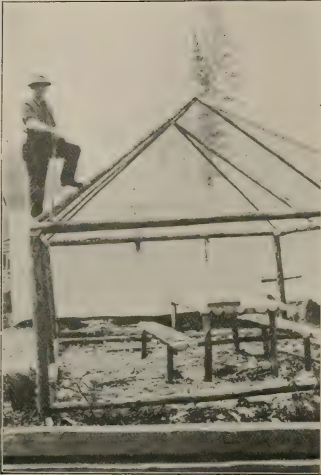
MR. MILLER AT 58-MILE, B. C., BUILDING THE FRAME OF THE READING TENT—NOTE TABLE MADE ENTIRELY OF POLES
