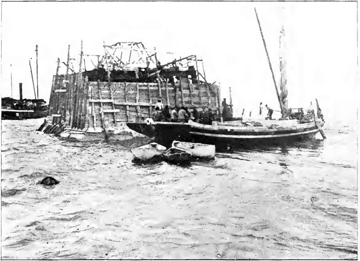
BEAUJEU BANK PIER, QUEBEC, UNDER CONSTRUCTION.
