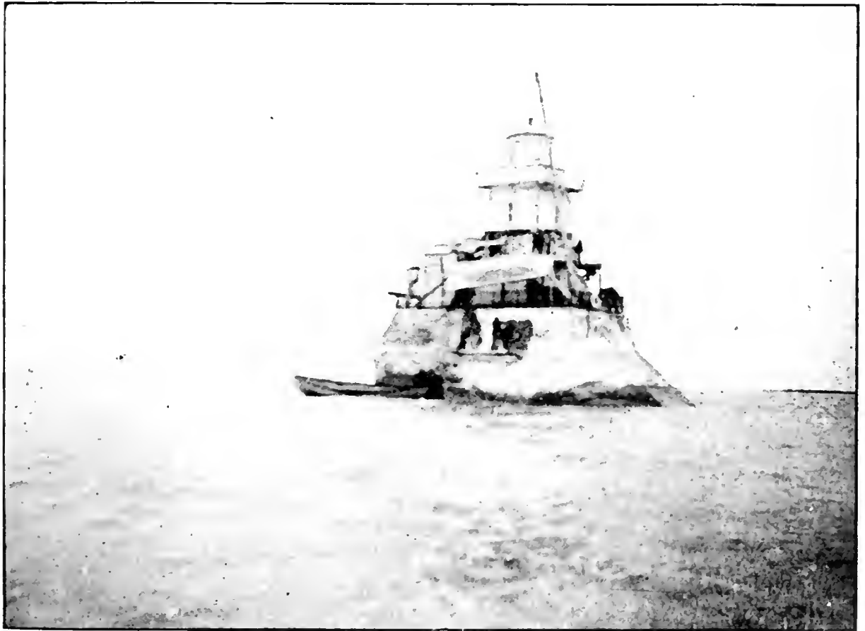
ALGERON ROCK LIGHTHOUSE, QUEBEC, UNDERGOING REPAIRS.
