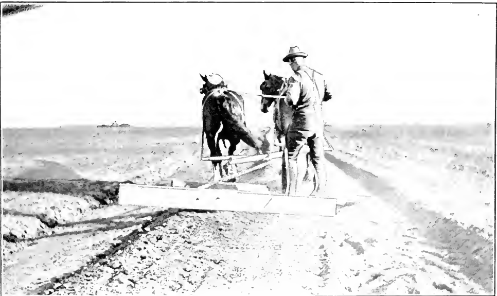
Grading Roads with the Split-log Drag, Experimental Station, Rosthern, Sask. 16—1913—p. 344
