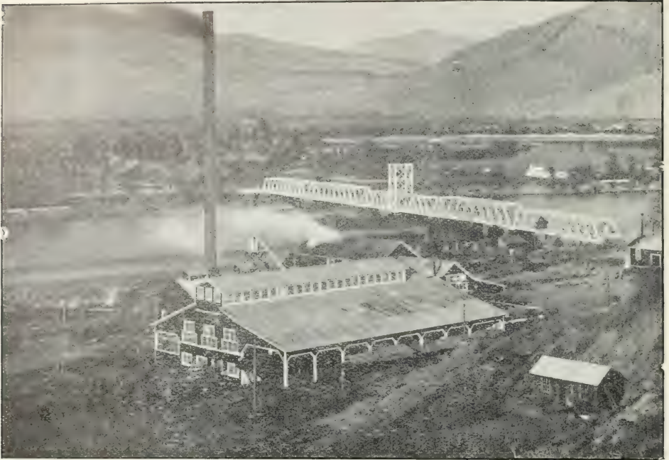
BRIDGE OVER THOMPSON RIVER AT KAMLOOPS
