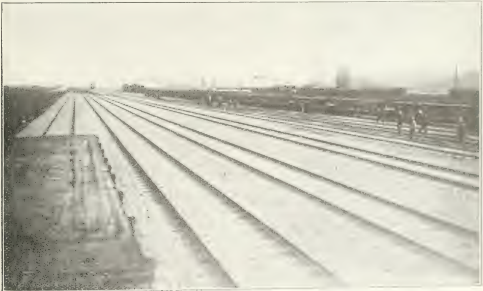
BUILDING THE GREAT C. P. R. TERMINALS AT COQUITLAM
