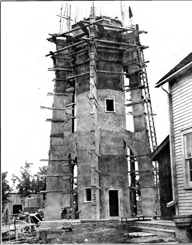
Caribou Island, Lake Superior, reinforced concrete lighthouse under construction.
