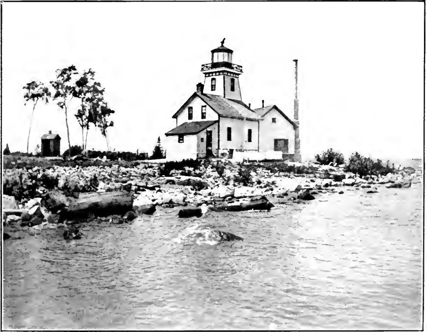
Hope Island Lightstation, Georgian Bay.
