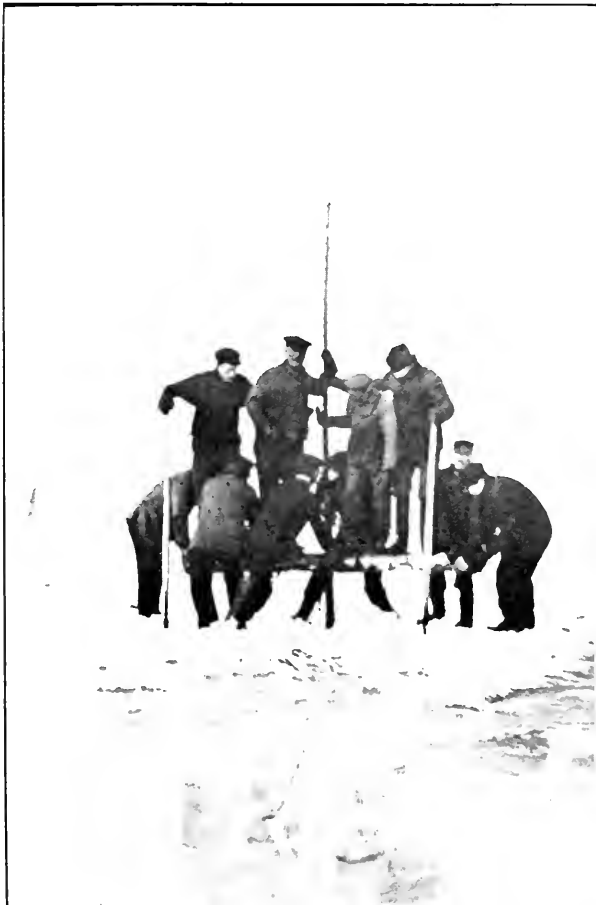
Showing method of putting in tamarac poles during the winter, to mark dredging limits on Lake St. Peter.
