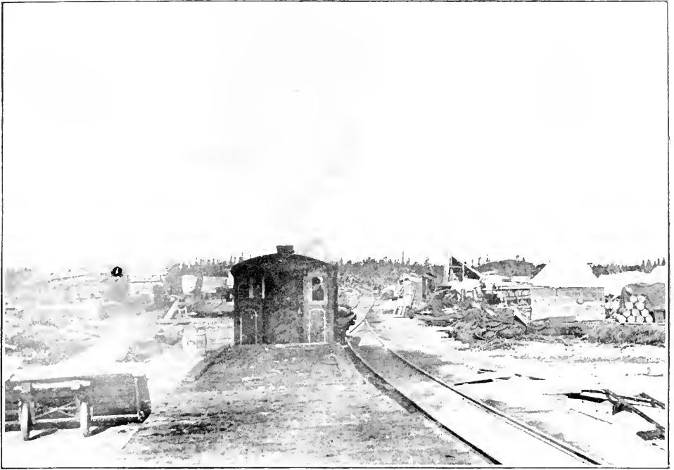
Hudson Bay Railway—Material yard, Port Nelson.
