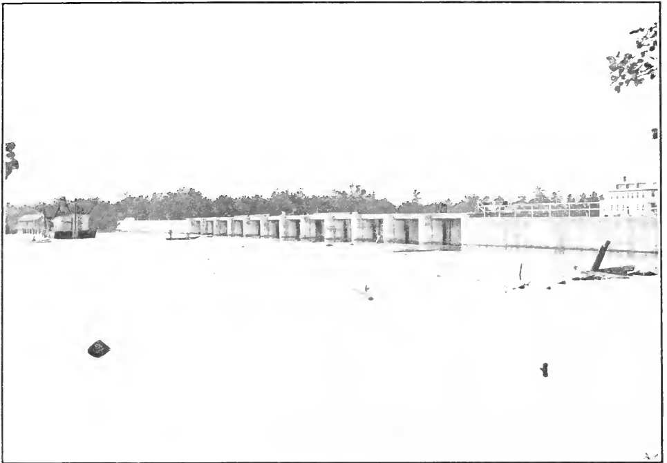
Trent Canal—Lakefield—Balsam Lake division. Up stream view of new Burleigh Falls dam.
