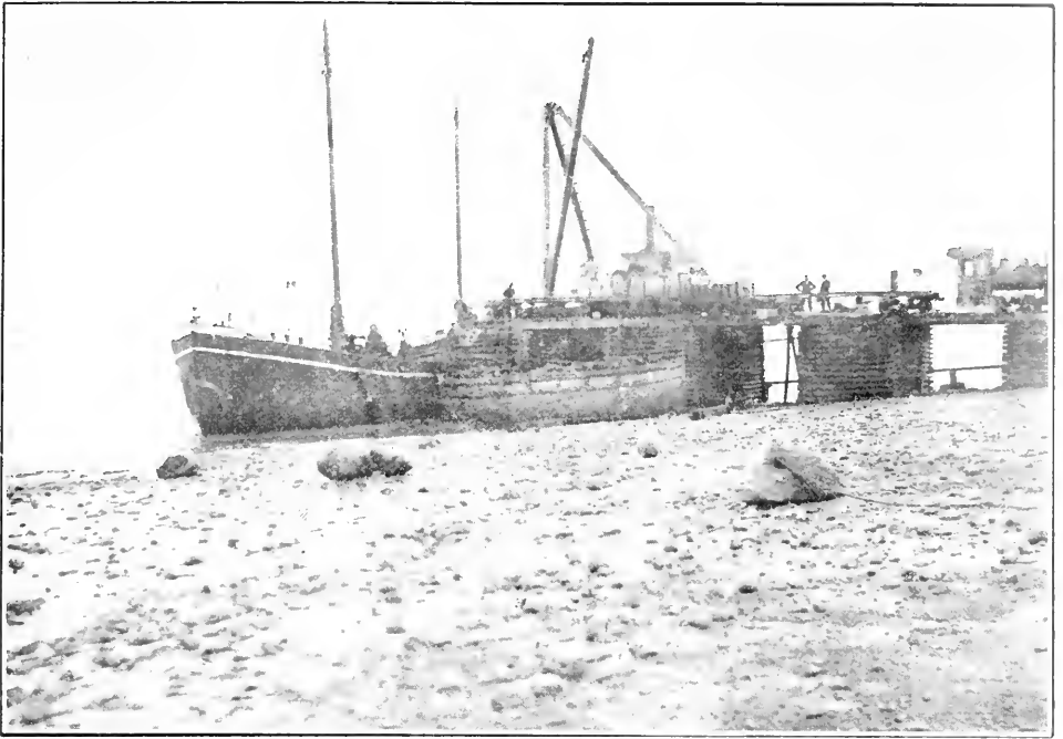
Hudson Bay Railway—Lighter at temporary wharf, Port Nelson.
