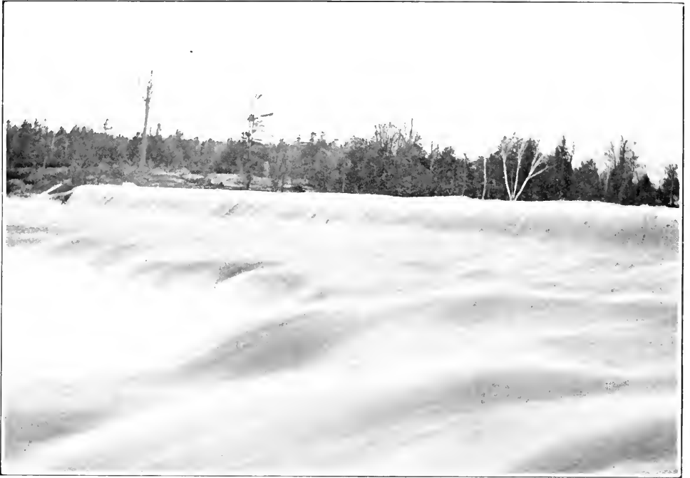
Trent Canal—Crow River Weir. Submerged dam.
