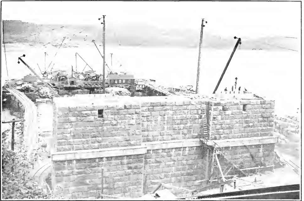
Quebec Bridge—North anchor pier and plant about north main pier.
