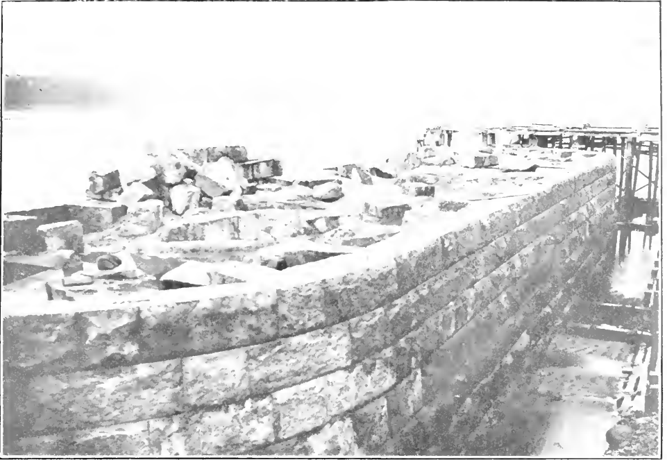
Quebec Bridge - North main pier in course of construction.
