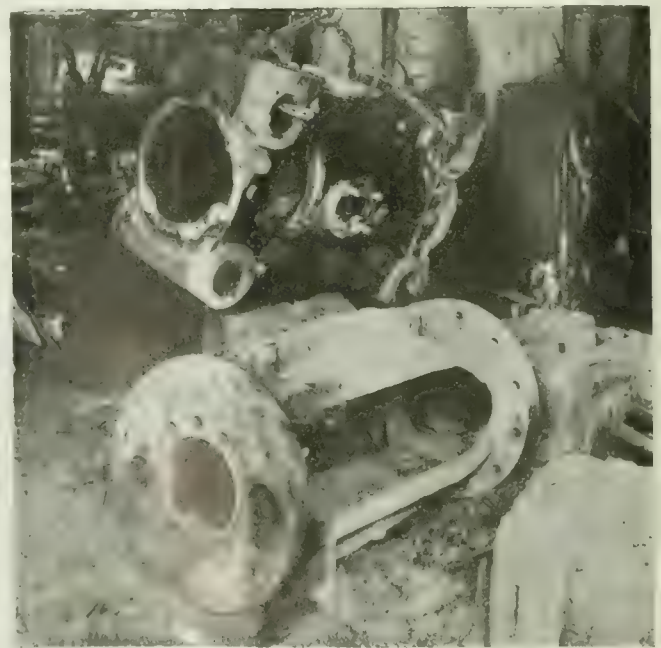
FIG. 5. SLIDE SHOWN IN FIG. 4. COMPLETELY REPAIRED. NOTE DAMAGED CYLINDER ABOVE WAITING REPAIR.
