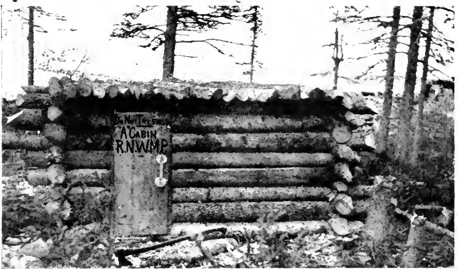
R.N.W.M. Police shelter cabin at Sulphur Point, Great Slave Lake, N.W.T.
