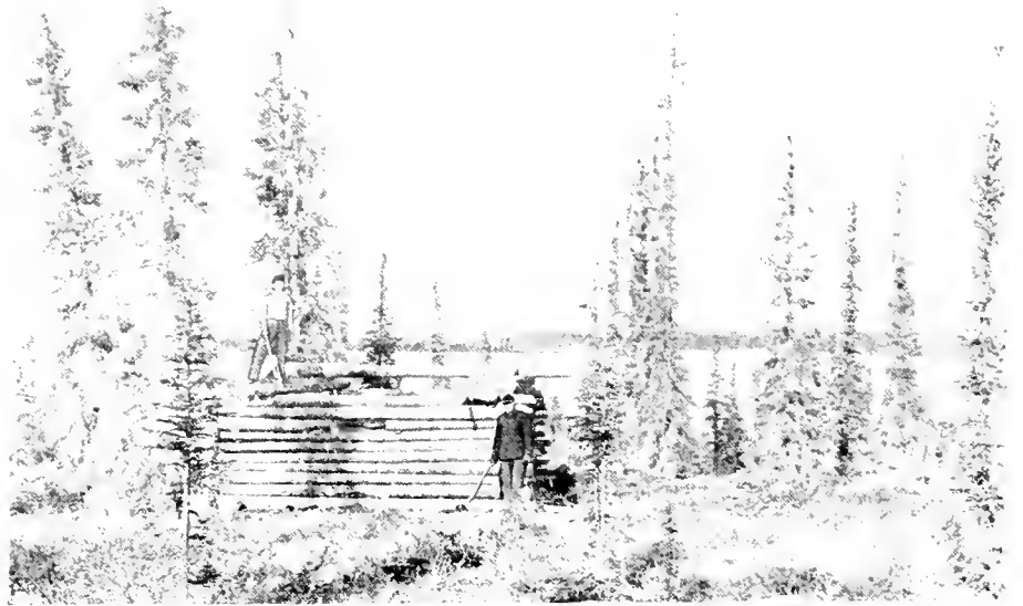
Constables Withers and Wight, building a storehouse, Dease Bay, N.W.T.
