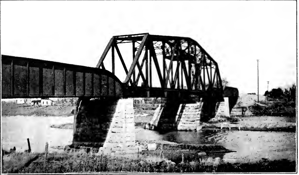
Assiniboine River, Headingly. Meter section at Bridge.
