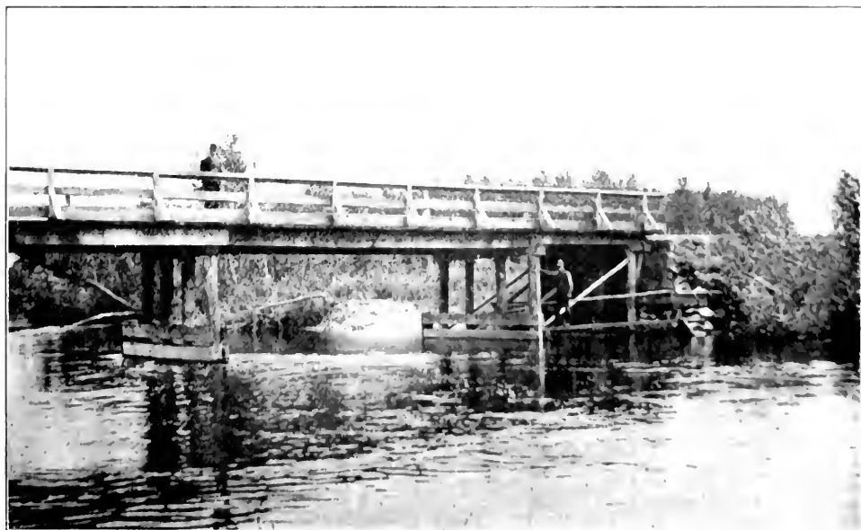
Brokenhead River, Simot. Bridge, showing gauge.
