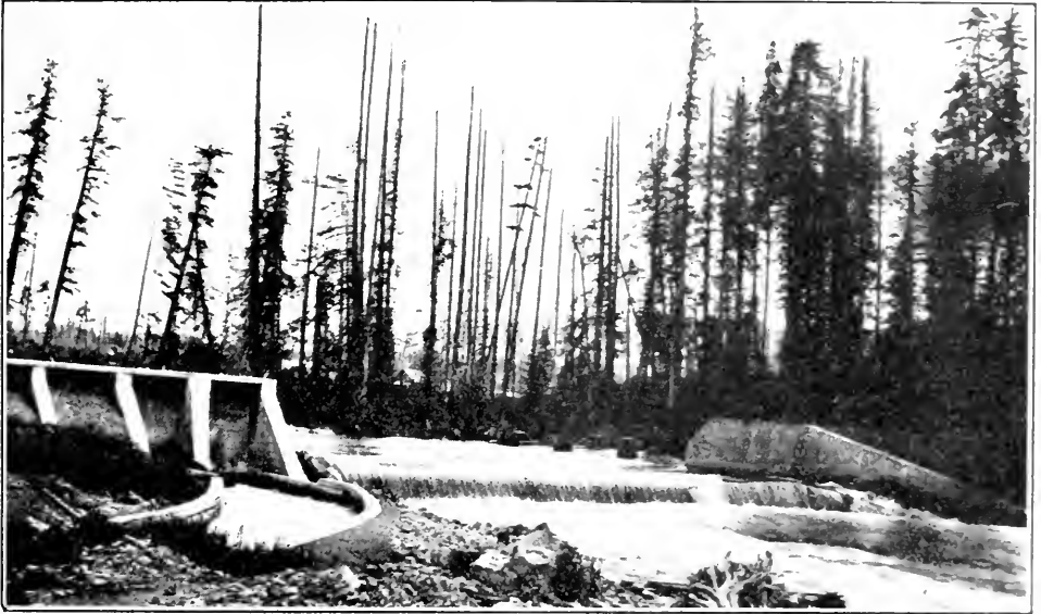
Diversion dam showing flume to intake, of Puntledge River Hydro-Electric Installation on Puntledge river about two miles below impounding dam.
