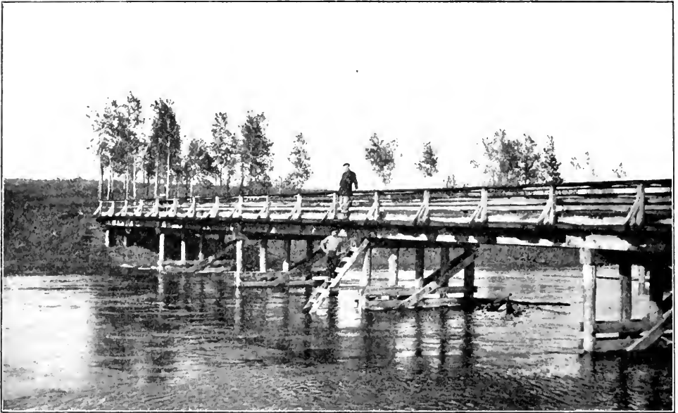
Whitemouth River at Whitemouth. Gauge at bridge.
