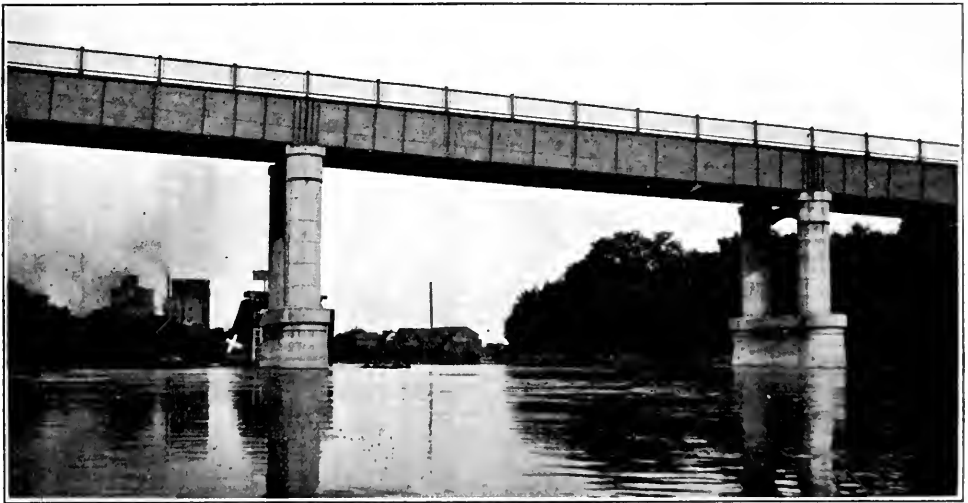
Assiniboine River, Brandon. Gauge at Bridge.
