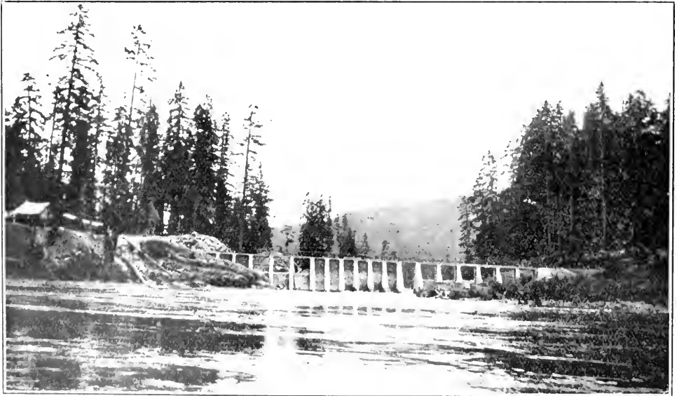
Impounding dam of Puntledge River Hydro-Electric Installation on Puntledge river near outlet from Comox lake.
