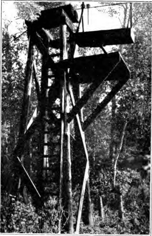
Cranbrook District (4E) Photograph showing support for cable way and platform attachment for cable car
