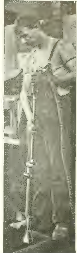
Sand Rammer in operation.
