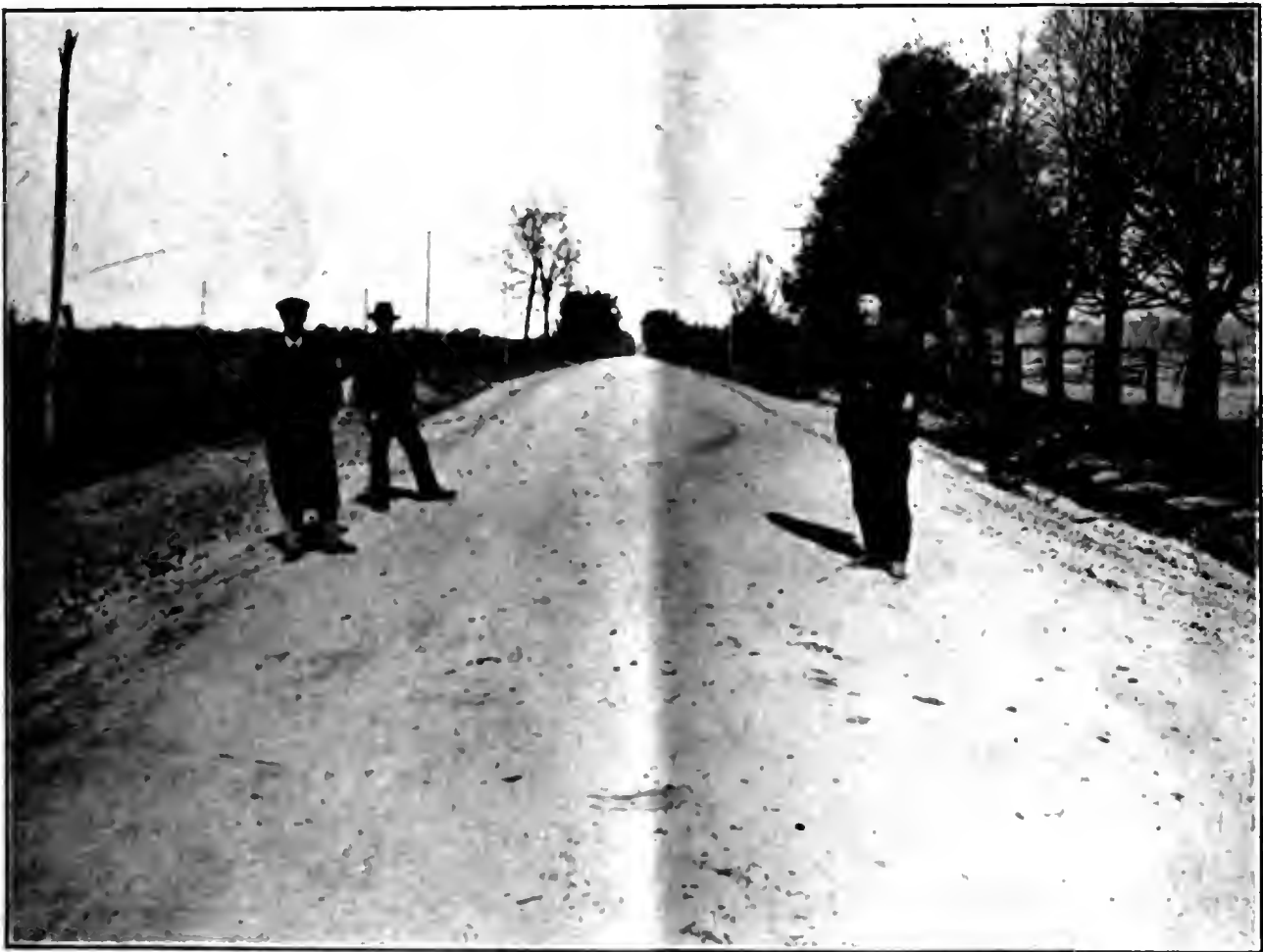
A completed Road in the County of Oxford
