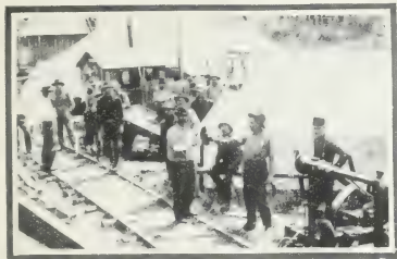
RAILWAYS LEAVE OPENINGS FOR CONSTRUCTION WORKERS
