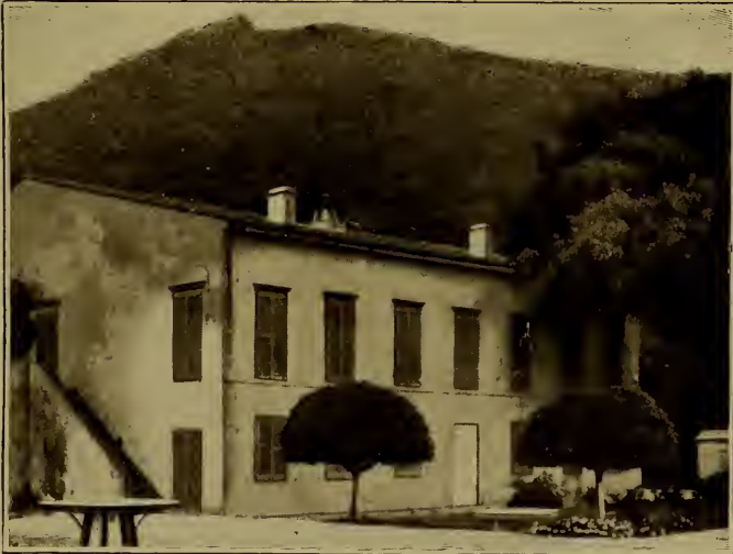
THE HOUSE AT SAN MARTINO, IN ITS ACTUAL STATE.
