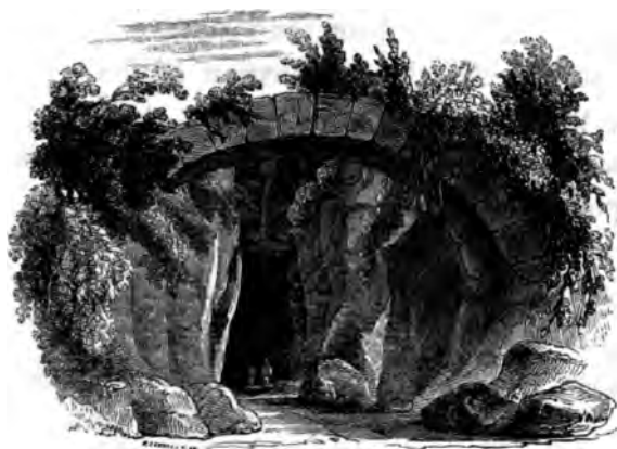
TUNNEL AT SELEUCIA.
