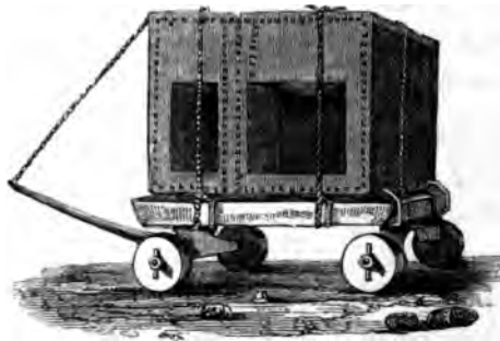
BOILER ON ITS WAGGON.
