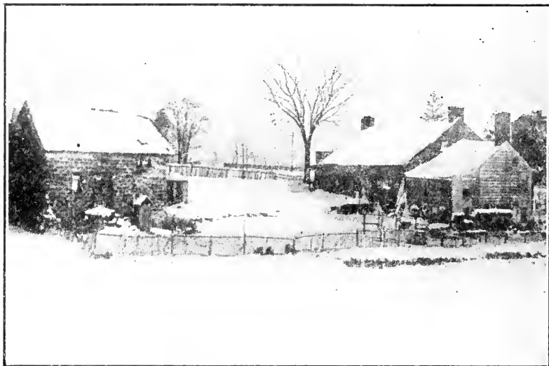
John Johnson Mill (about 1700) on former site of City Almshouse, Elizabeth Avenue
