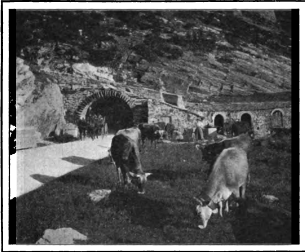
The Kaltwasser Cascade Tunnel,
