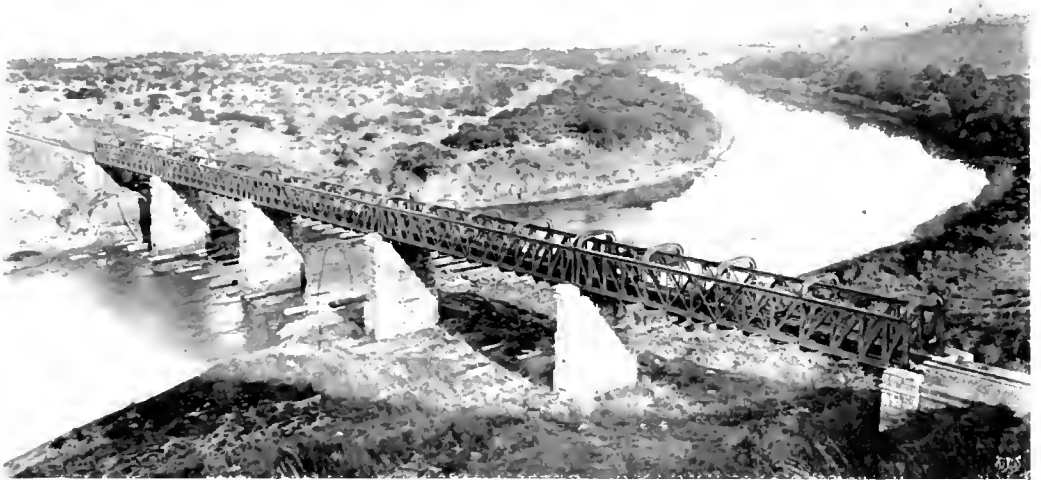
NEW RAILWAY BRIDGE AT COLENZO (FROM FORT WYLIE)
