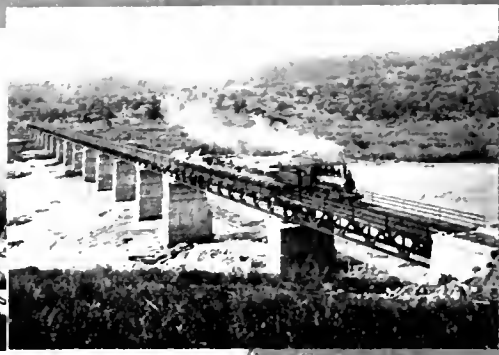
Lower Tugela Bridge
