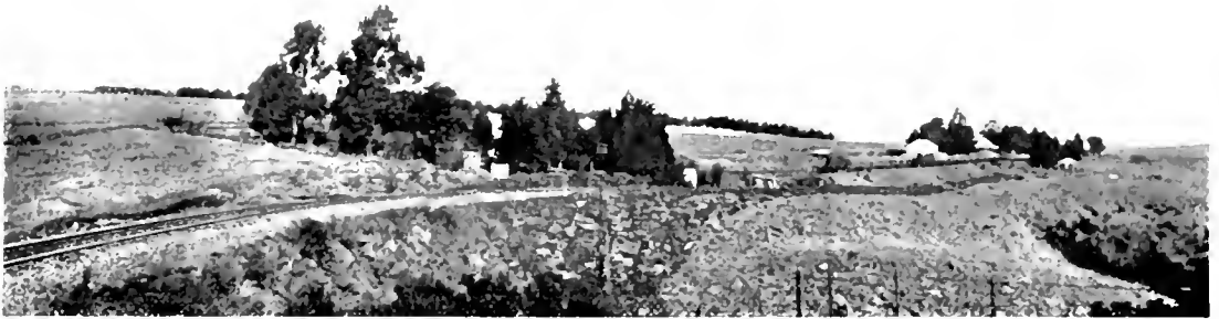
HIGHLANDS STATION, 5,000 FEET ABOVE SEA LEVEL
