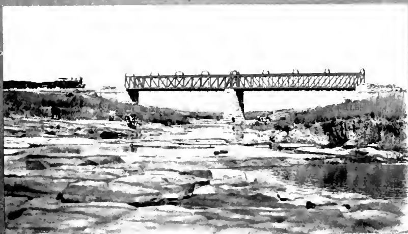
Railway Bridge Frere
