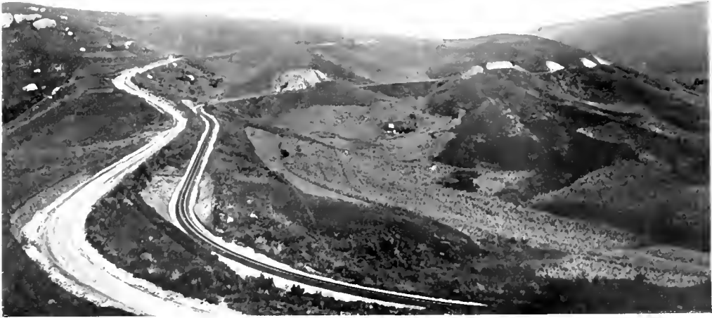
BY RAIL AND ROAD, NEAR BOTHA'S HILL
