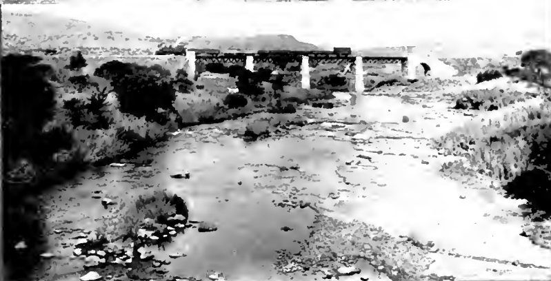
Railway Bridge over Bushman's River. Estcourt
