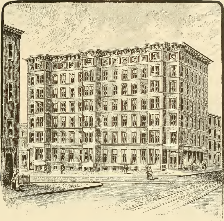
THE W. B. MOSES BUILDING.
