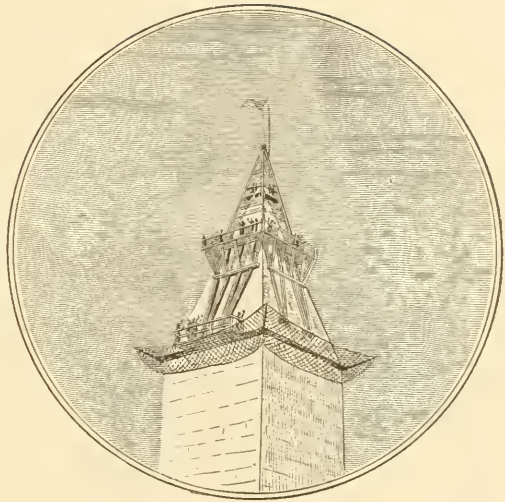
STAGING AT THE TOP OF THE MONUMENT DURING THE WORK OF COMPLETION.
