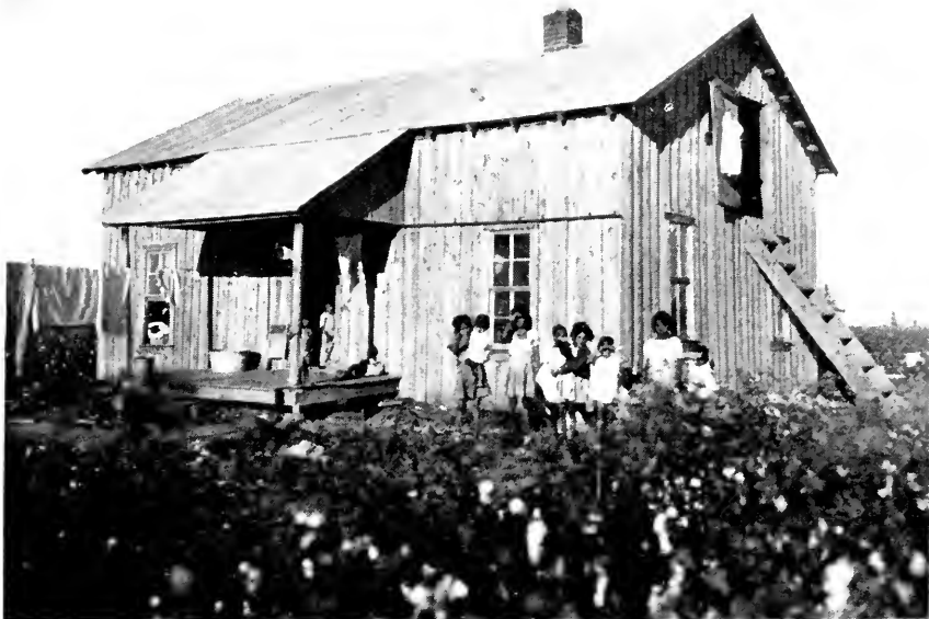
House used by migratory Mexican cotton pickers. Several families from Hidalgo County, Tex., used this house. Men slept in the attic reached by the outdoor stairs.
