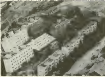
Earthquake-induced ground failure (liquefaction) can endanger even the most well-constructed buildings (Niigata, Japan, 1964).
