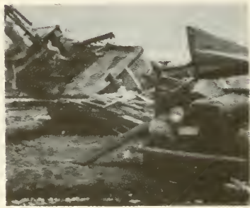
Valdez, Alaska, waterfront after tsunami caused by 1964 Good Friday earthquake.
