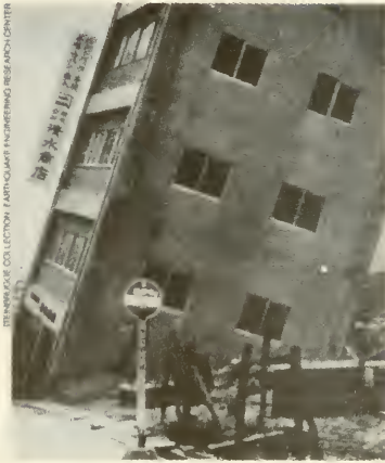
Failure of the ground itself can make an otherwise sound building unusable.
