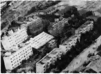
Earthquake-induced ground failure (liquefaction) can endanger even the most well-constructed buildings (Niigata, Japan, 1964).
