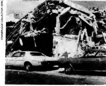
Many older buildings are vulnerable to structural collapse
