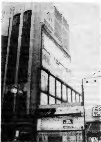
An unexpected side-effect of the Los Angeles seismic retrofit program was the partial demolition and conversion of multistory buildings into low, single-story structures
