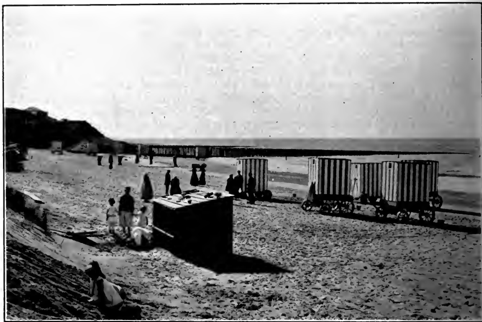
Pile Dikes for Protection against Marine Erosion
