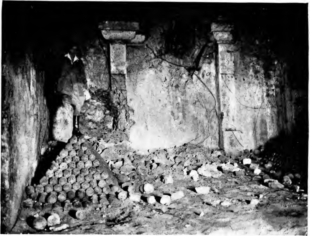
HOLES DUG IN THE WALLS OF CHRISTOPHE'S CITADEL IN SEARCH OF TREASURE
