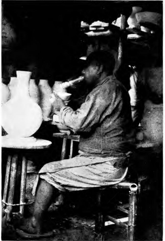
ONE METHOD OF APPLYING PORCELAIN GLAZE
