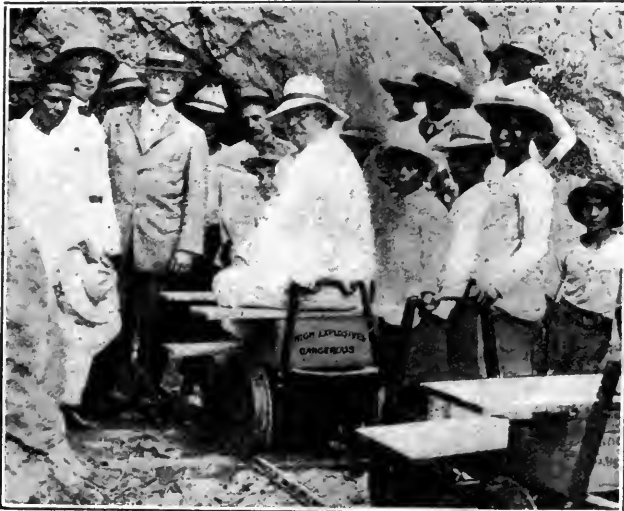
THROUGH THE AQUEDUCT ON A HAND CAR
