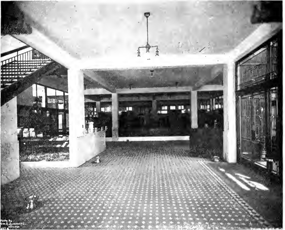
CORRIDOR OF THE ARMOUR OFFICES
