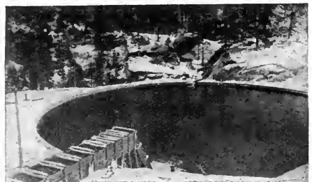
RE-ENFORCED CONCRETE SETTLER AT HEAD OF PIPE LINE Pike's Peak Hydro-Electric Company
