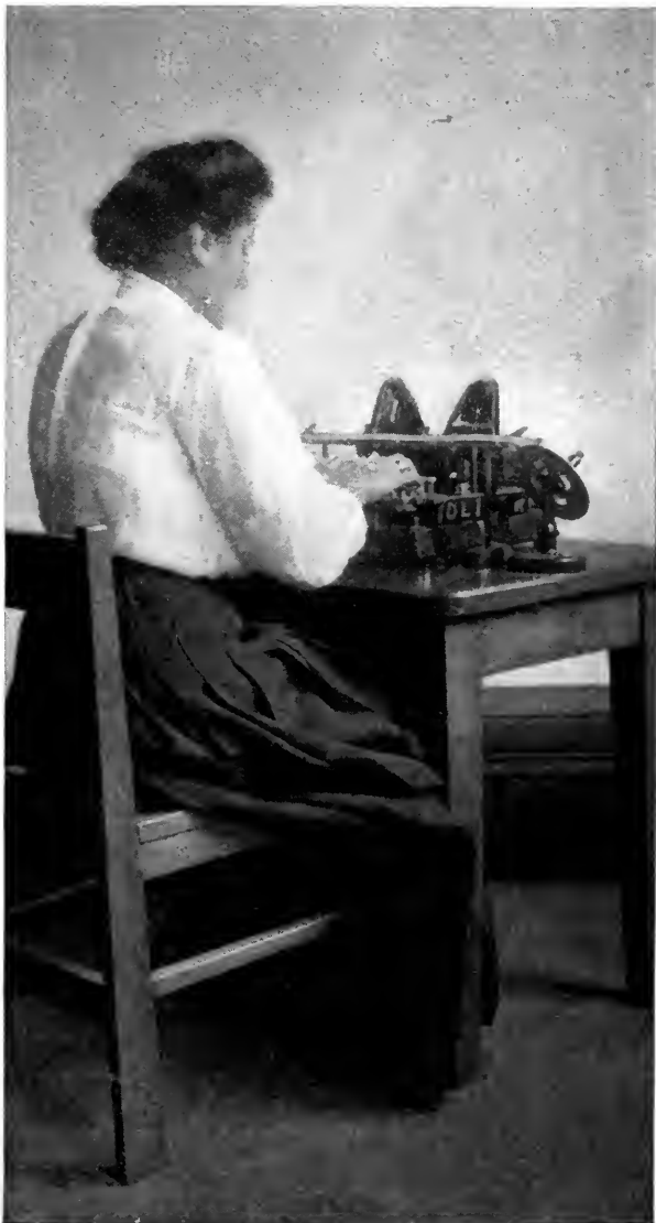
TRANSCRIBING A TELEPOST MESSAGE—CHEMICALLY RECORDED IN MORSE CHARACTERS
