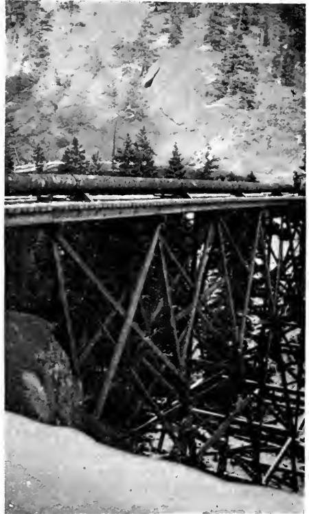
SCENE ALONG THE PIPE LINE Pike's Peak Hydro-Electric Company
