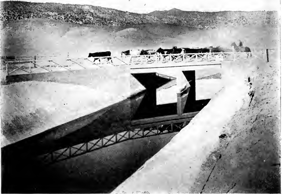
CONCRETE BRIDGE AND LINED CONDUIT, KERN RIVER PLANT OF THE PACIFIC LIGHT AND POWER COMPANY
