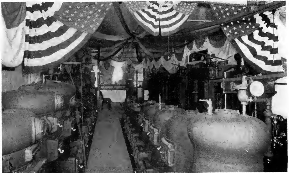
A GLIMPSE OF THE COUNTING ROOM THROUGH A VISTA OF MODERN HEATERS
