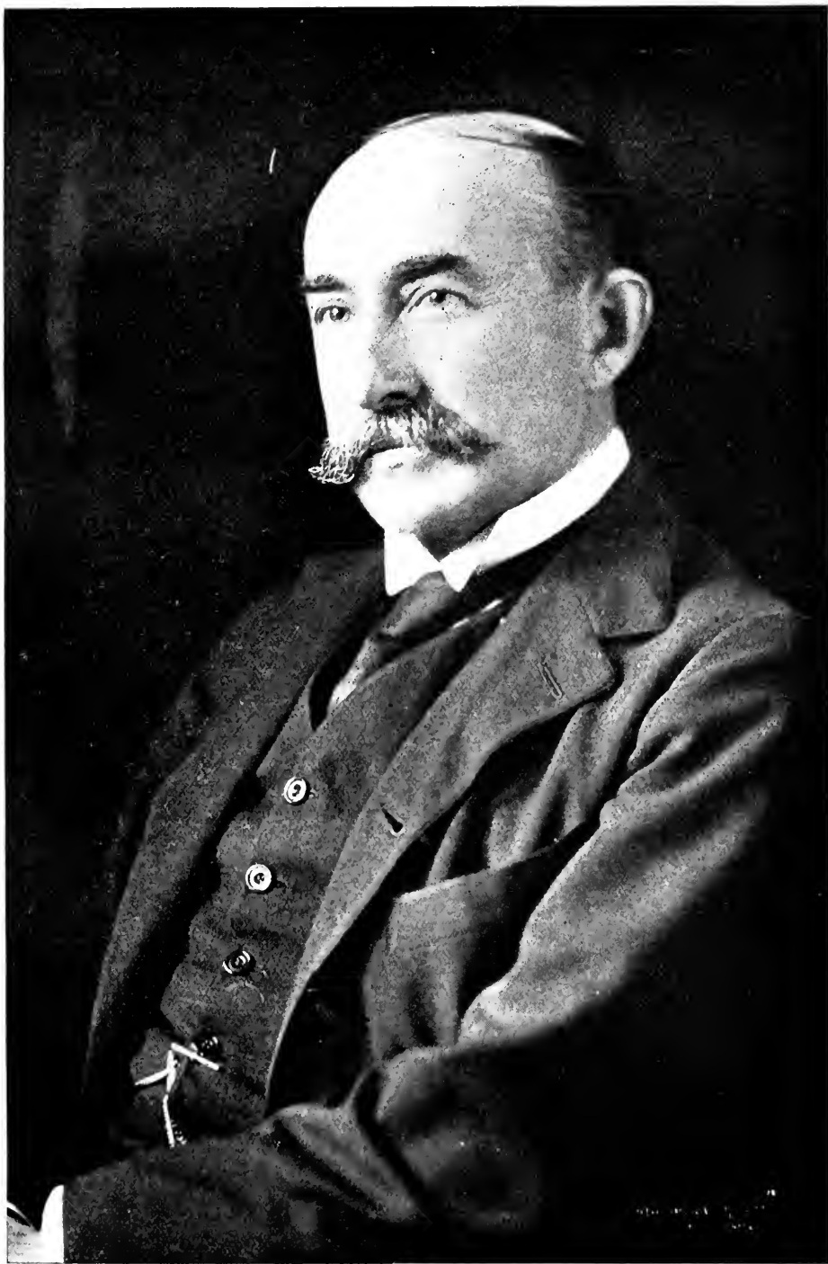
JOHN HAYES HAMMOND, THE NOTED MINING ENGINEER
