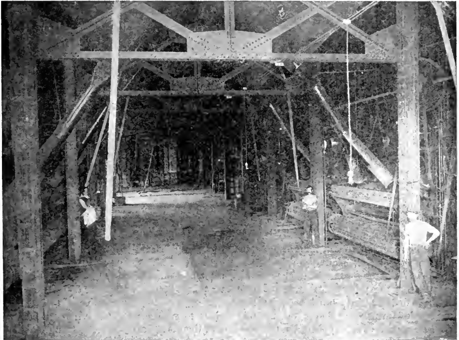
BOILER ROOM, SHOWING STOKERS—PEOPLE'S POWER CO. PLANT, MOLINE, ILL.
