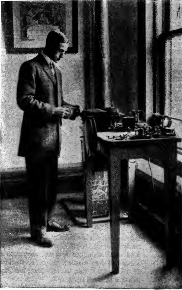
REMOVING THE REEL OF TELEPOST MESSAGES RECEIVED AT 1,000 WORDS A MINUTE
