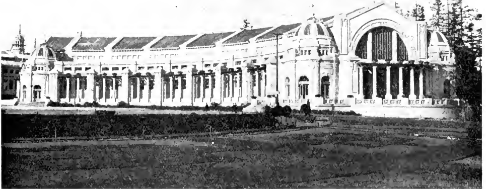
MANUFACTURES BUILDING. ALASKA-YUKON-PACIFIC EXPOSITION
