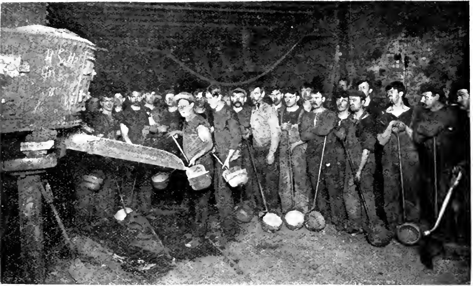
ONE OF THE GREAT CUPOLAS — THE HUSKY POURERS WITH CRUCIBLE LADIES WAITING THEIR TURN
