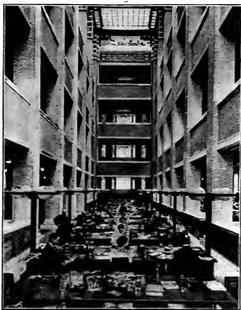
The central court, Larkin Administration Building
