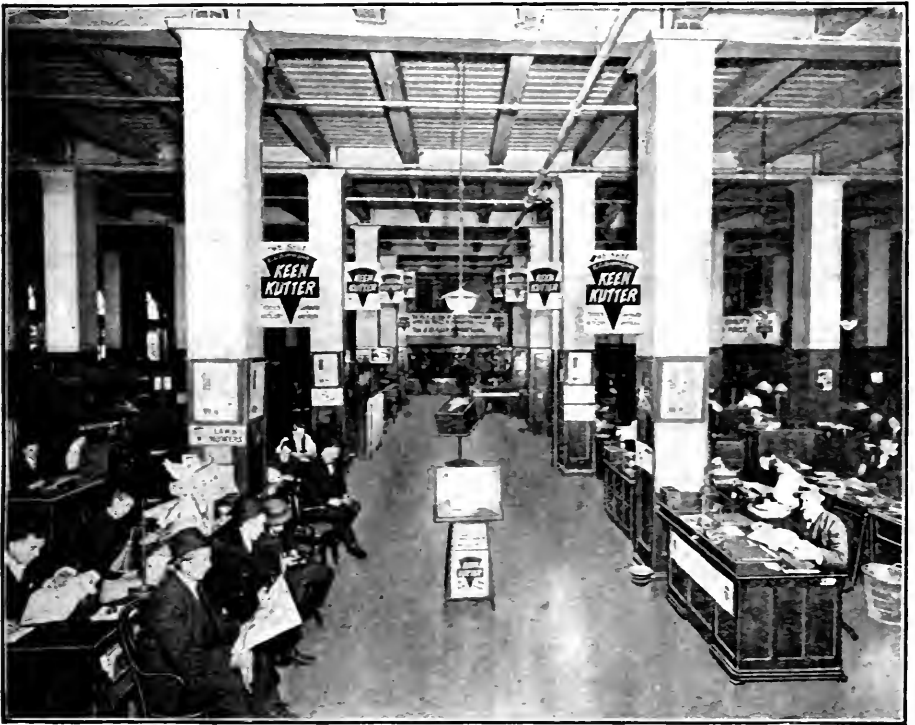
Entrance to general offices
