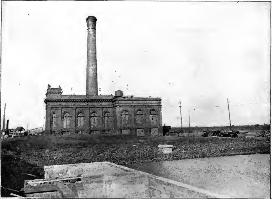
NEW POWER HOUSE AT BELLE ISLE Oklahoma Railway Company
