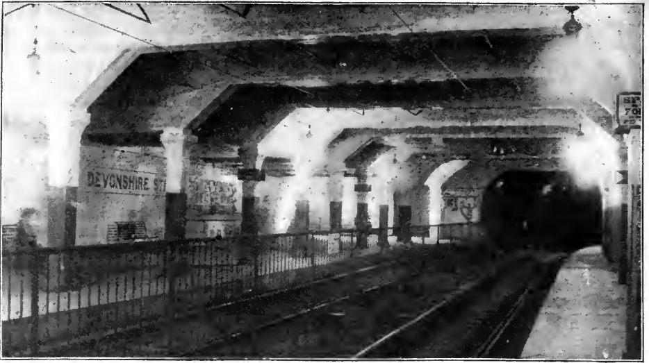
DEVONSHIRE STREET STATION, EAST BOSTON TUNNEL.
