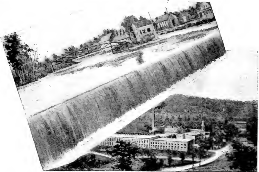
1. The Walden factory; employs 535 skilled workmen, where "Keen Kutter" pocket knives are made. 2. Water power. Water power is used for both factories. 3. Location of "Keen Kutter" tool factory among New Hampshire Hills
