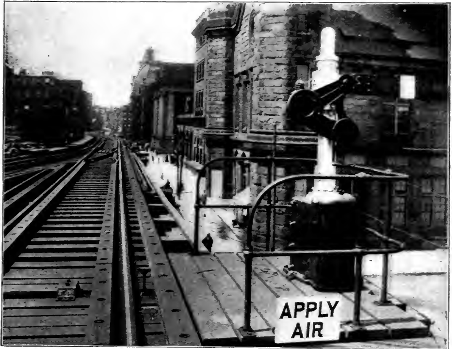
SEMAPHORE SIGNAL AND AUTOMATIC TRIP FOR AIR BRAKES
