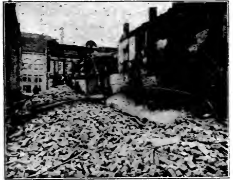
Ruins of a business block, Hartford City, Indiana, wrecked by a gas explosion. Four persons were buried in the debris, and the ruins presented a very peculiar appearance, each brick standing out separate, the mortar having apparently disappeared in the explosion.—Mabel Morehead.
