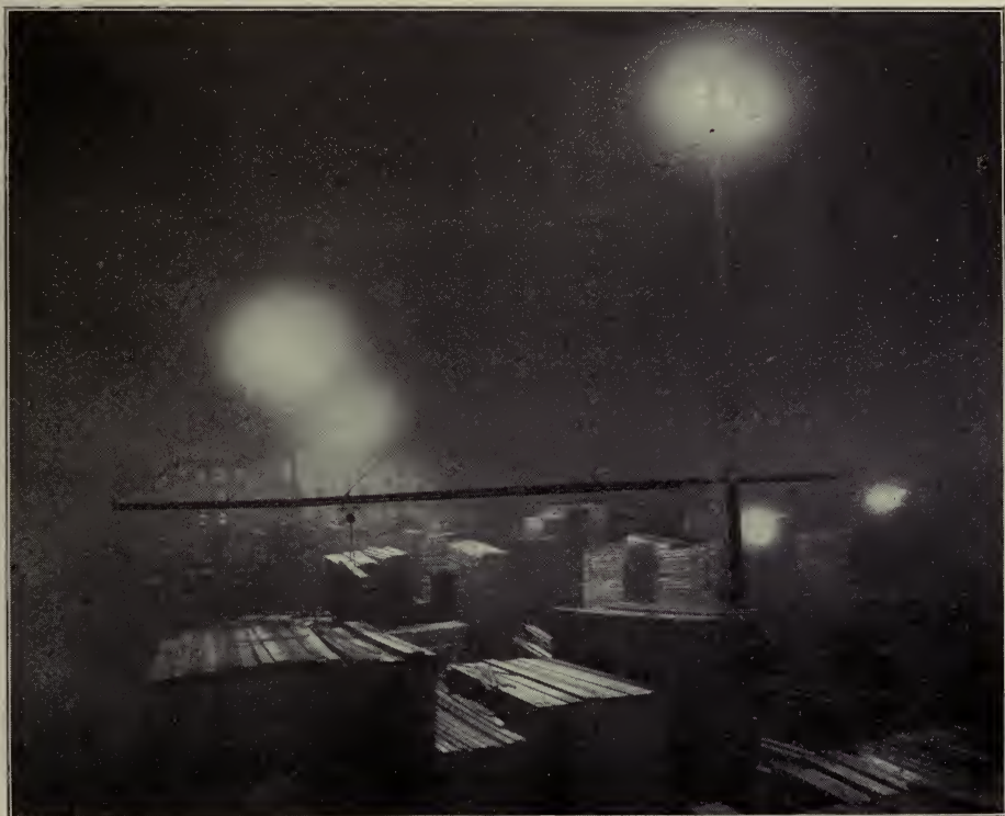
THORNTON-CLANEY LUMBER COMPANY'S YARD Flaming arcs for night work and motor driven cranes
