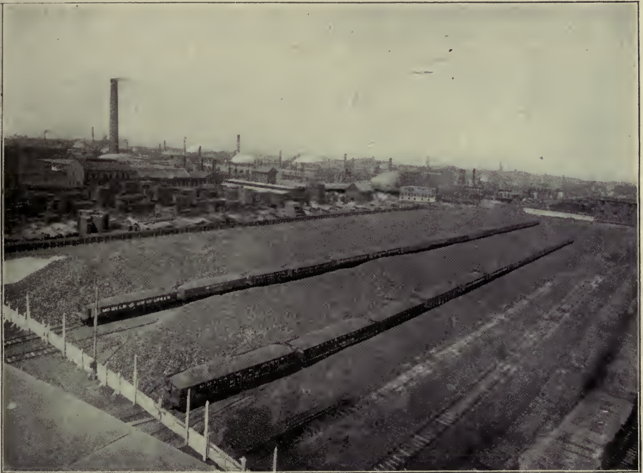
SECTION OF COAL STORAGE IN YARDS OF THE FISK STREET POWER HOUSE
