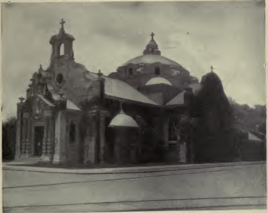
CHRIST EPISCOPAL CHURCH, PENSACOLA
