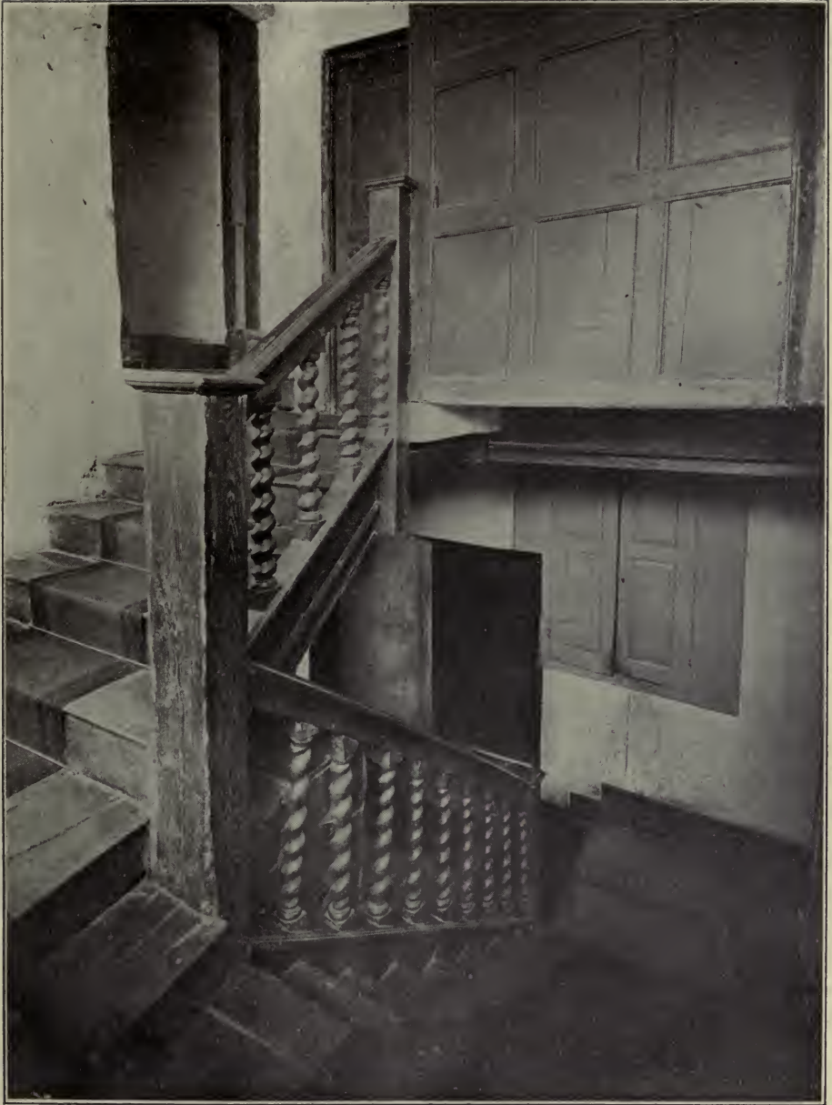
OAK STAIRCASE, SULGRAVE MANOR
