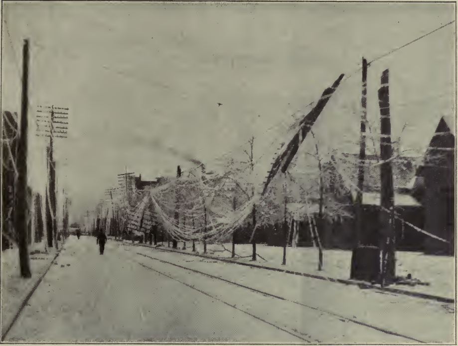
SLEET PULLING THE WIRES DOWN
