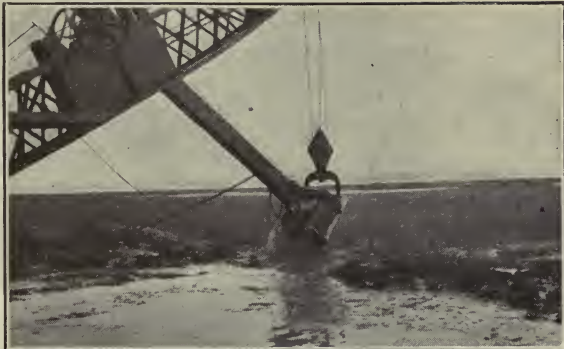
Dredge cutting canal
