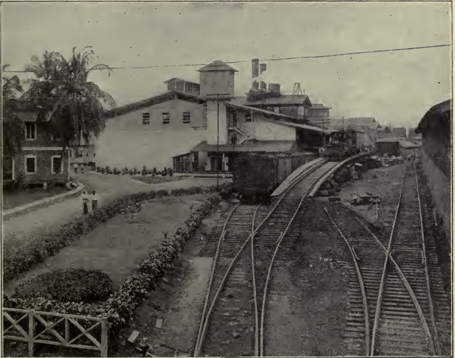
COLD STORAGE PLANT AT COLON WHERE THEY STORE EATABLES
