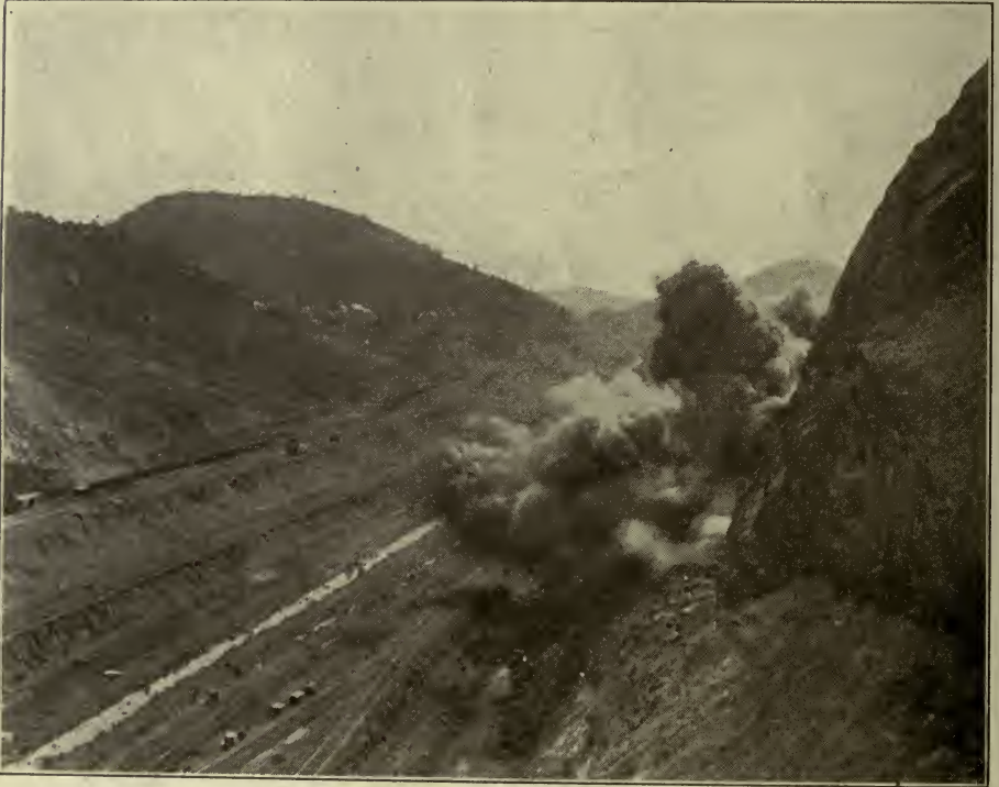
CULEBRA CUT AT CULEBRA, BLASTING ROCK ON CONTRACTOR'S HILL, VIEW LOOKING SOUTH
