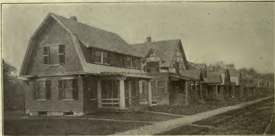
TYPE OF AMERICAN WOOLEN COMPANY'S DETACHED COTTAGES For operatives at Lawrence, Massachusetts. Six rooms, bath and pantry. Rents at $4.15 per week
