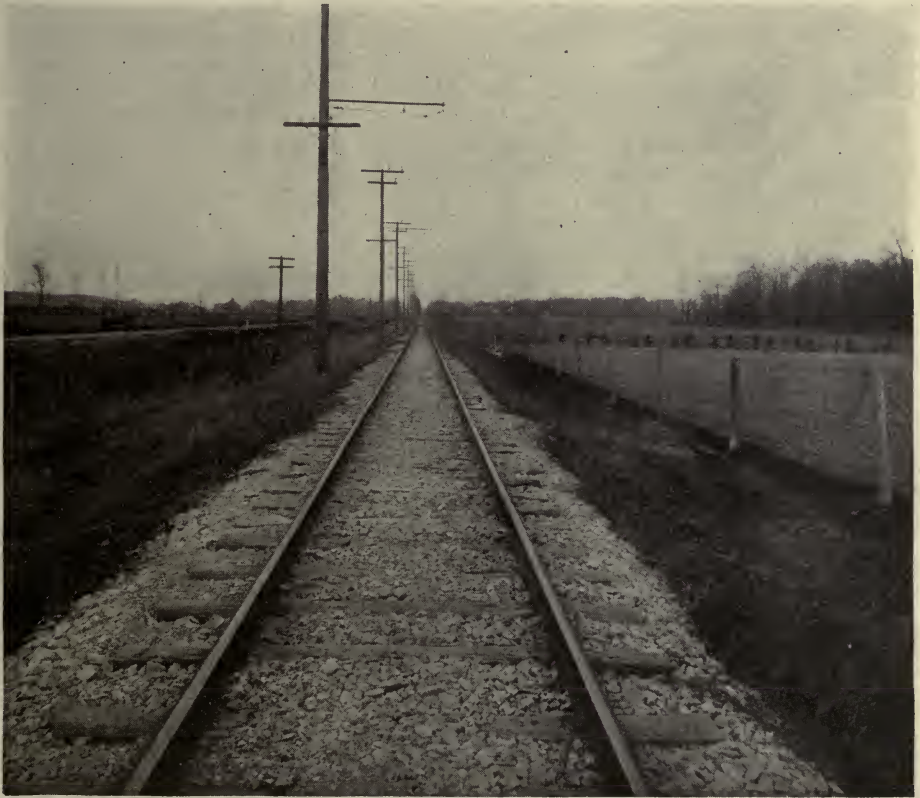
VIEW OF INTERURBAN ROADWAY
