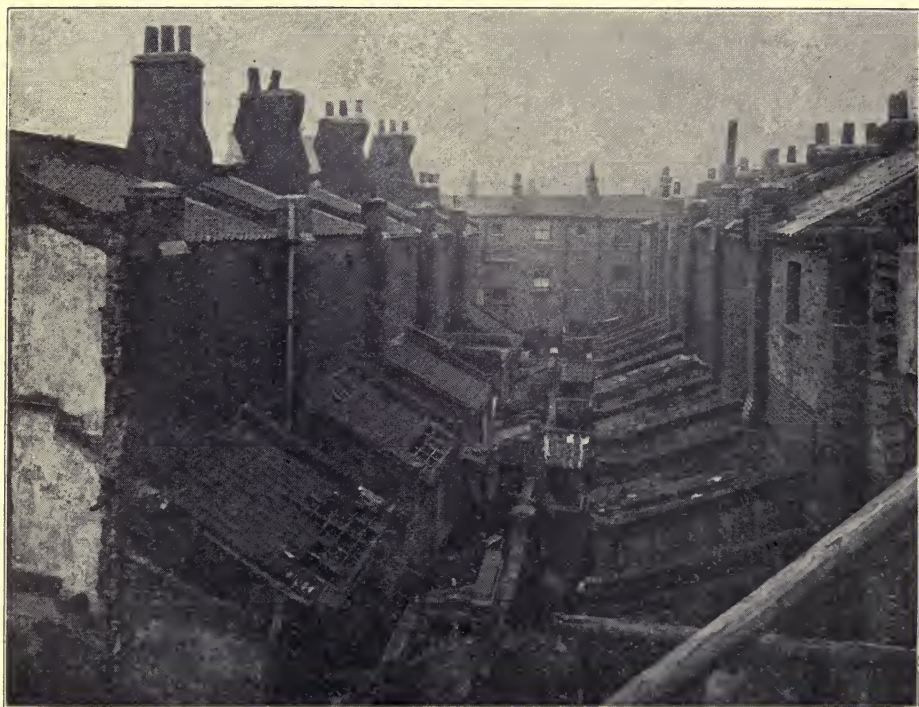
BELL LANE AREA BEFORE SLUM CLEARANCE
