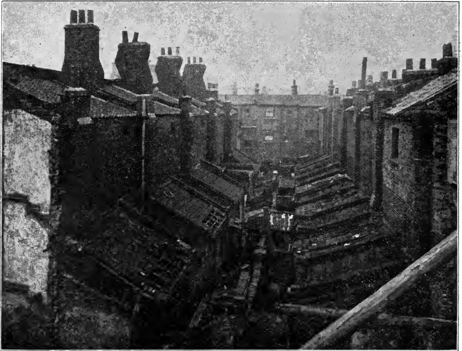
BELL LANE AREA BEFORE SLUM CLEARANCE
