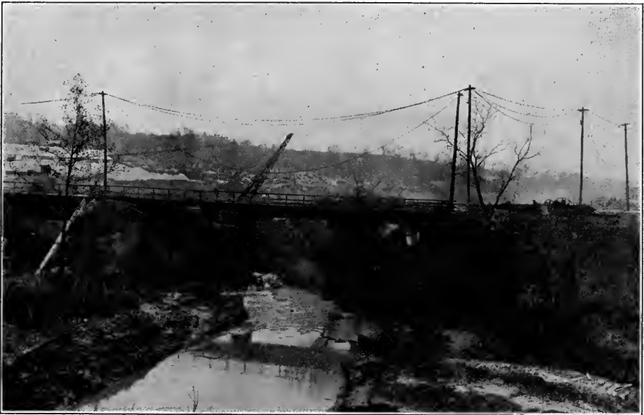
RIVER DES PERES BEFORE IMPROVEMENT
