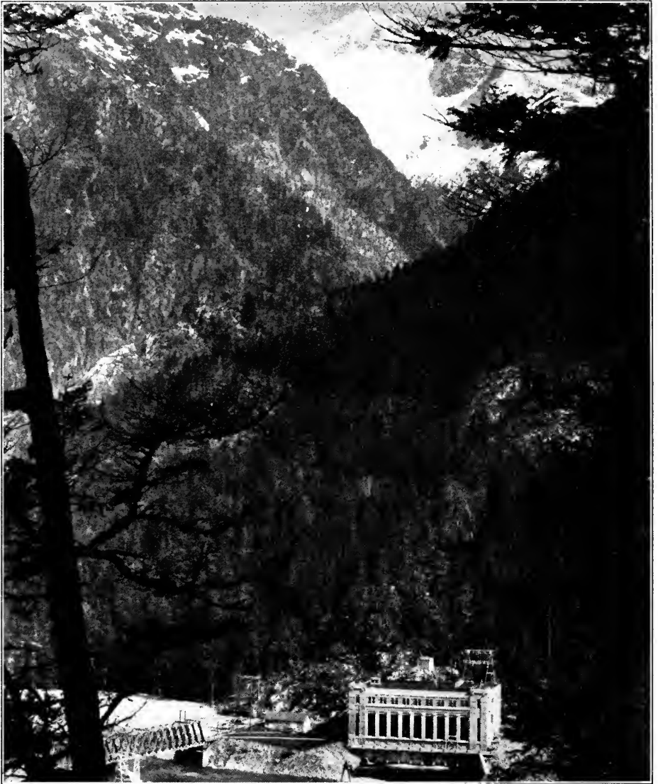
GORGE POWER HOUSE—SEATTLE MUNICIPAL SYSTEM
