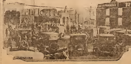
View of the ruins of Mexia, Tex., after the recent conflagration which caused a damage of nearly a million dollars. The town sprung up almost overnight as the result of oil discoveries, and it will be rebuilt as rapidly as is possible.
