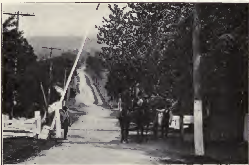
A VIEW FROM OUT OF THE PAST—CHARACTERISTIC TOLL BARRIER AND STRONG CORD REACHING ACROSS TO THE HOUSE ON THE RIGHT—HAND SIDE OF THE ROAD; ALSO KEEPER IN THE ACT OF COLLECTING TOLL.
