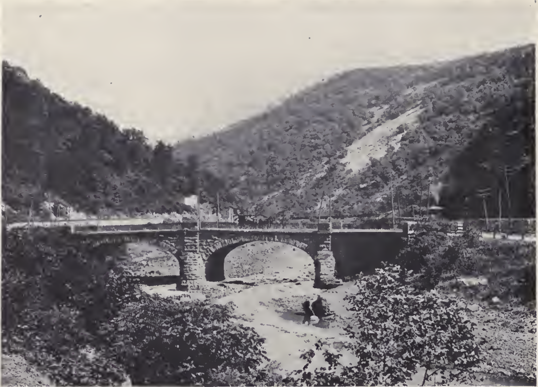
CLOSE VIEW OF THE HISTORIC STONE BRIDGE OVER WILLS CREEK, IN THE "NARROWS," A SHORT DISTANCE WEST OF CUMBERLAND, MD.
