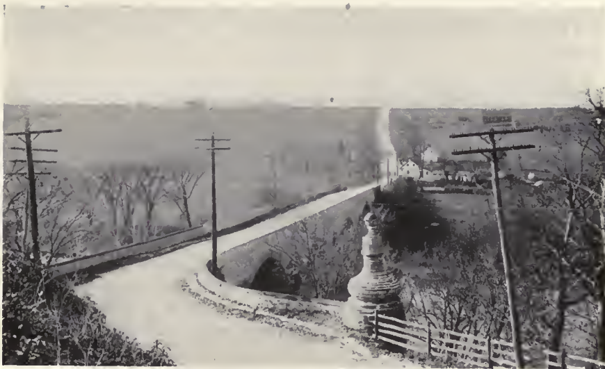
OLD STONE BRIDGE OVER THE MONOCACY RIVER, ABOUT THREE MILES EAST OF FREDERICK, MD.
