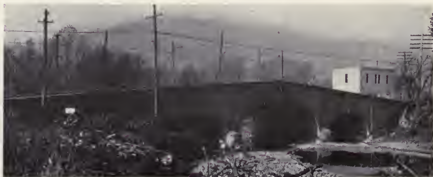
Photograph Copyright J. K. Lacock THREE-ARCHED STONE BRIDGE OVER LITTLE WHEELING CREEK AT ELM GROVE, W. VA., ABOUT FIVE MILES EAST OF WHEELING
