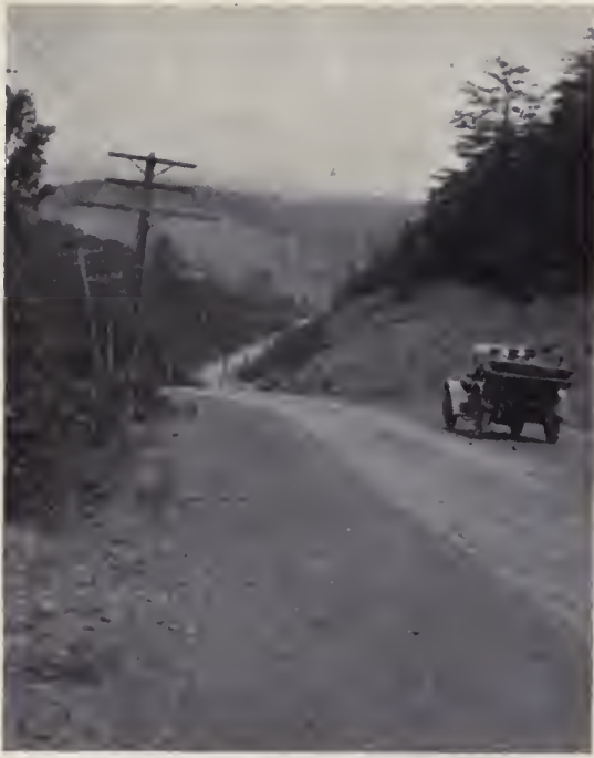
ROADWAY IN MARYLAND, NEAR THE FOOT OF GREEN RIDGE
