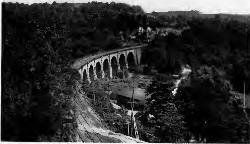
VIEW OF THE B. & O. R. R. BRIDGE OVER THE PATAPSCO RIVER, AND STATION, RELAY, MARYLAND, LOOKING NORTHEAST
