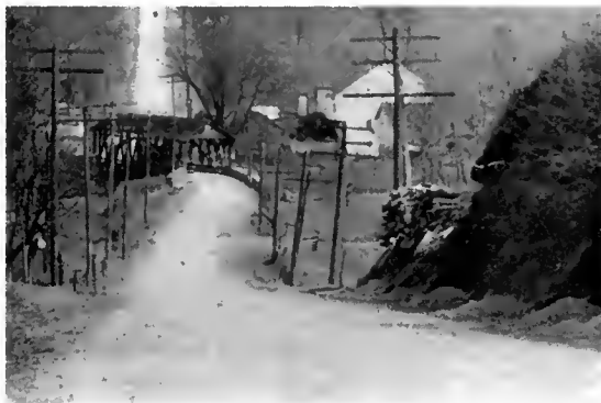
OLD COVERED BRIDGE JUST WEST OF MIDDLETOWN, MARYLAND. NOTE THE STEEP RISE OF THE PIKE BEYOND
