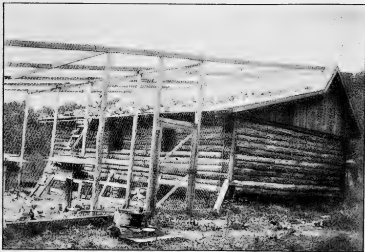
SQUAB HOUSE BUILT OF LOGS.
