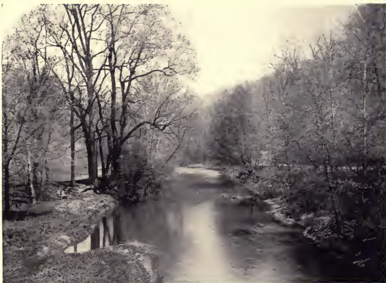
VIEW FROM KLINGLE ROAD BRIDGE
