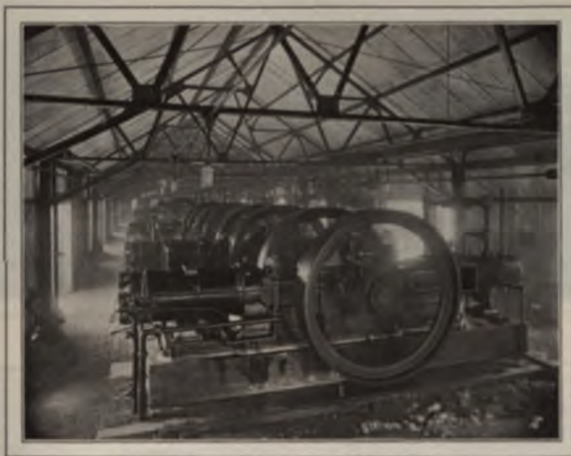
RIVERSIDE-WESTERN OIL COMPANY'S GASOLINE PLANT NO. 4.
