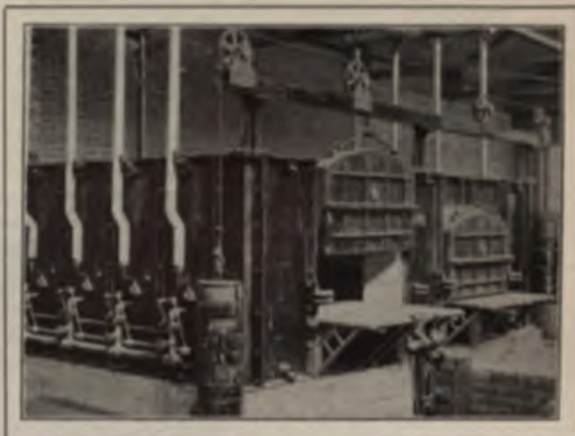
FIG. 6. COMBINATION OIL & GAS HEATING FURNACE.
