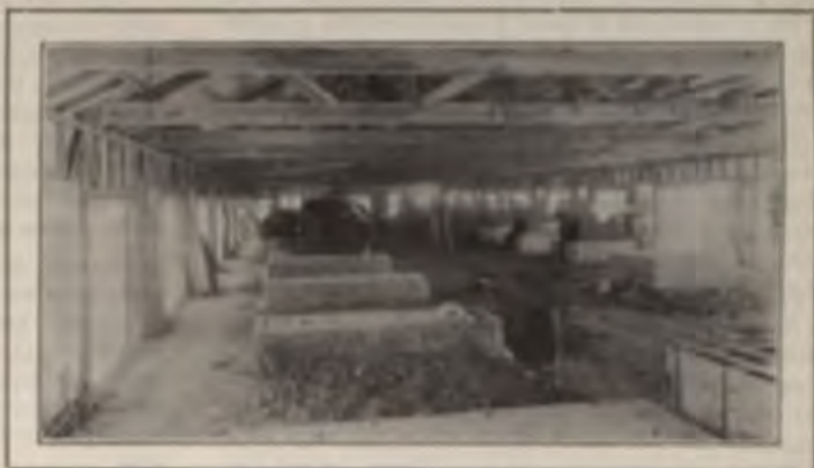
INTERIOR VIEW OF GASOLINE PLANT NO. 1 OF RIVERSIDE WESTERN OIL COMPANY.
