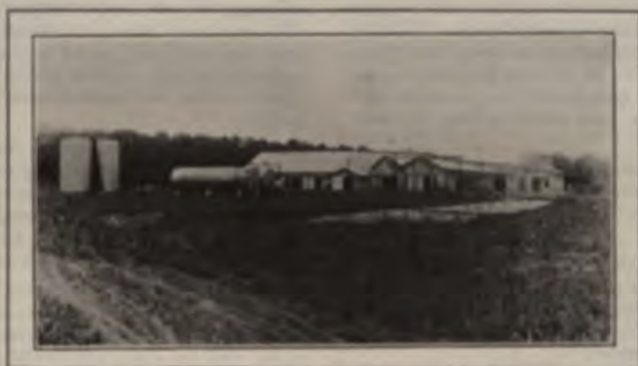
RIVERSIDE-WESTERN OIL COMPANY'S PLANT NO. 2
