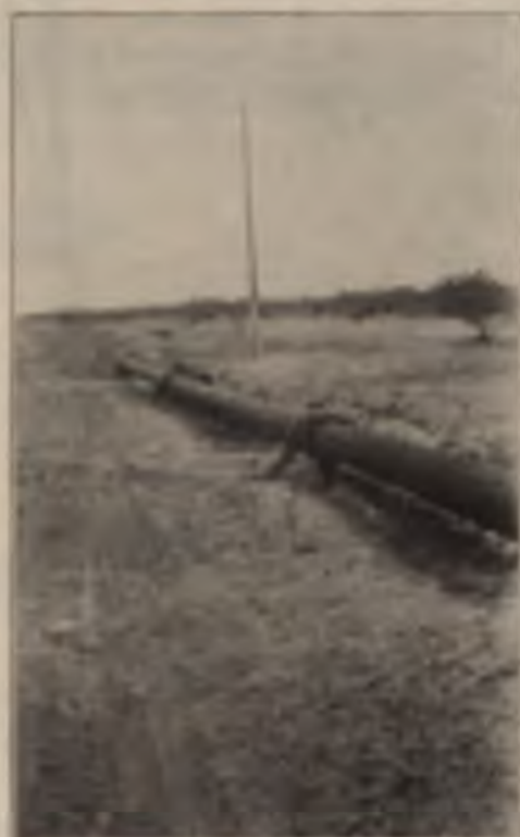
PIPE COUPLER SUPPORTS.
