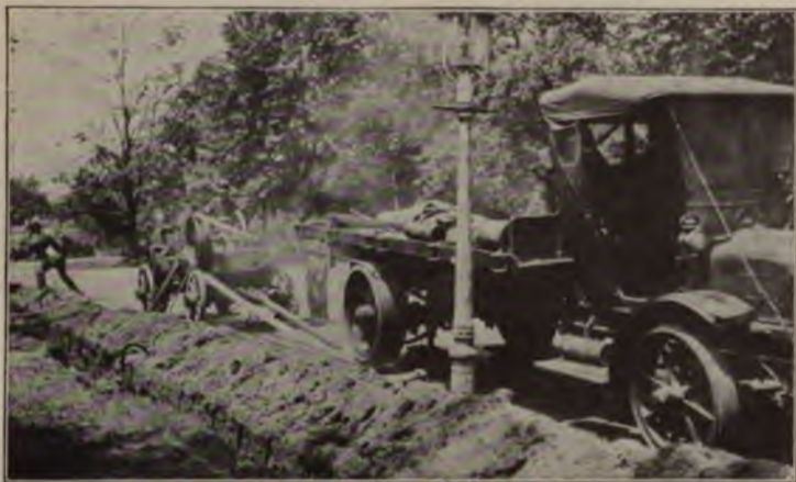
TESTING WELDED SECTIONS.
