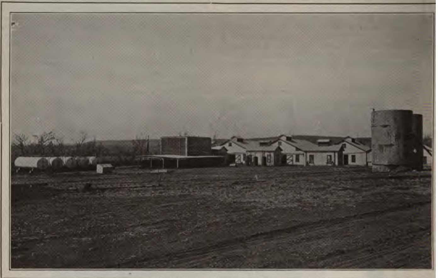
NO. 4 PLANT OF RIVERSIDE-WESTERN OIL CO. NINE MILES WEST OF DELAWARE, OKLA.
