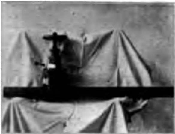
FIG. 1. A simple and inexpensive method of sealing a small gate valve. It is made of fabric or tarpaulin.
