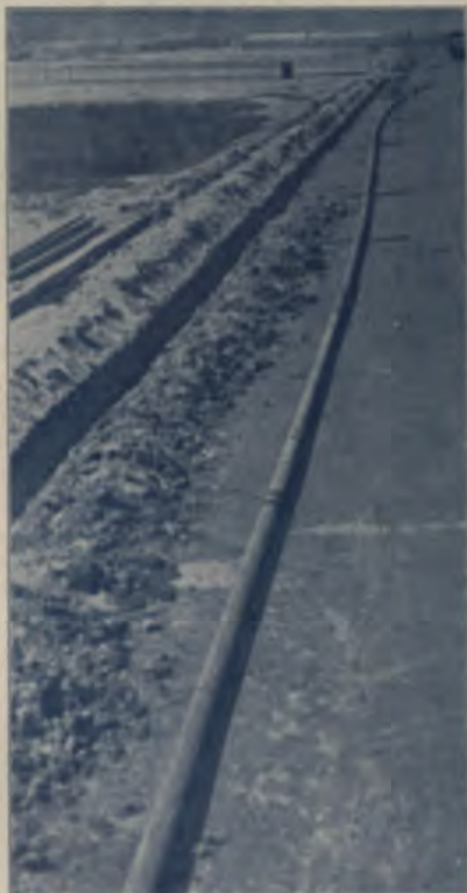
NOTE THE FLEXIBILITY OF A WELDED GAS LINE — Ready to Lay.
