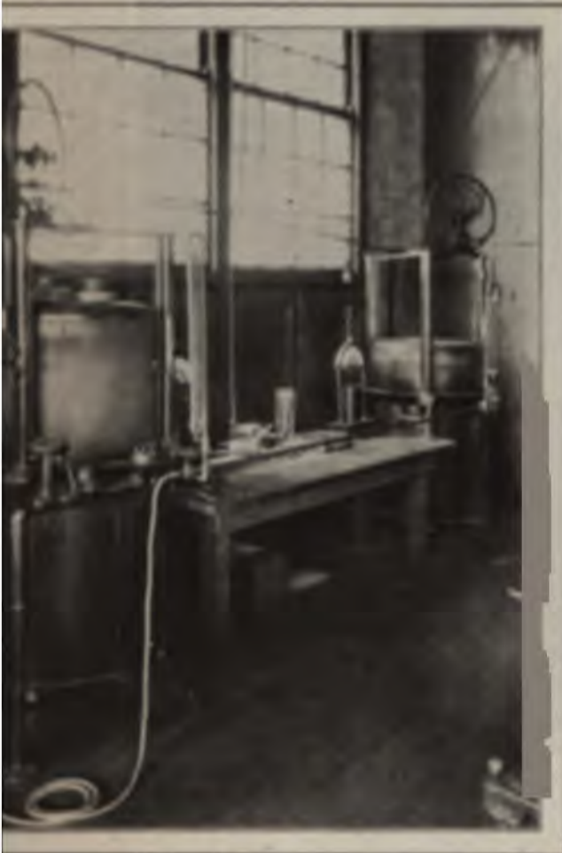
ARRANGEMENT OF METERS AND REGULATORS.
