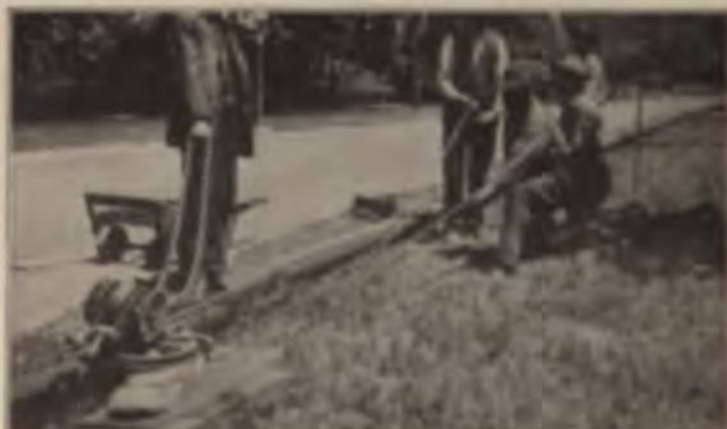
APPARATUS FOR DRAWING TOGETHER WELDED SECTIONS.
