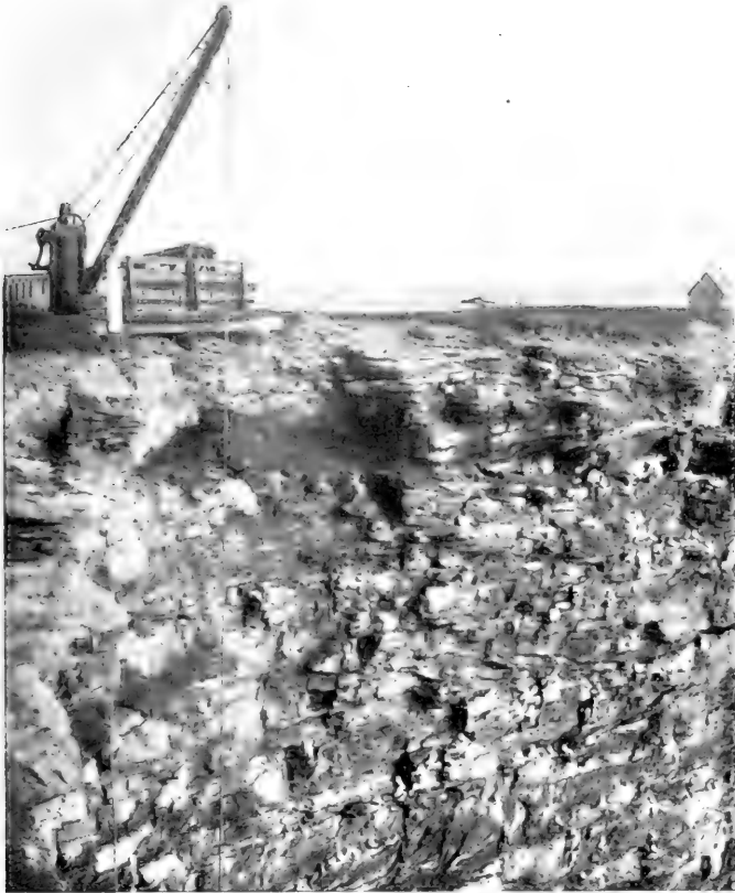
THE LANDING ON TOP OF THE ROCK, SHOWING CRANE.
