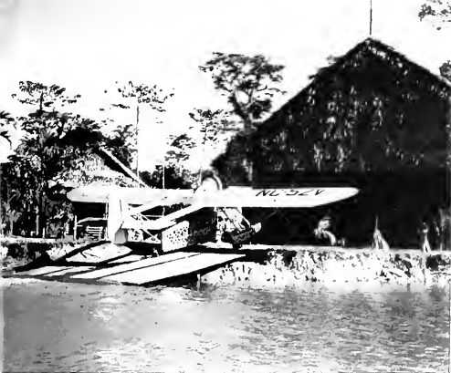
(Above) A GRASS HANGAR was built to protect the plane from the almost incessant rains. The ramp of ironwood was constantly being devoured by tiny insects and had to be repaired repeatedly. To the left of the hangar stands the dining room
