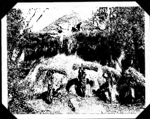
MARTIN JOHNSON'S PHOTOGRAPHIC LABORATORY under construction: part of the 'village' that sprang up around the Johnsons' home near beautiful Lake Paradise, where they passed some of the happiest years of their life
