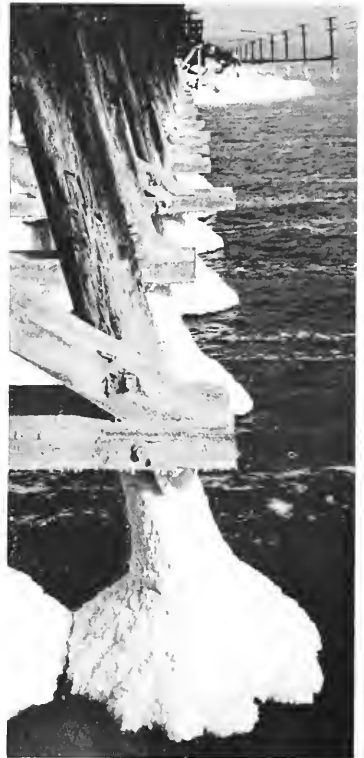
SALT ACCUMULATIONS on pillars in Great Salt Lake, Utah. The crust is 18 inches thick at the water line
