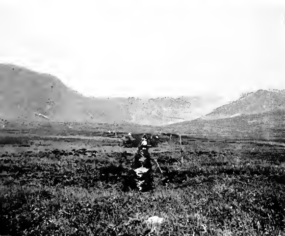
THE DIGGING of a draining ditch through a bog at Narssak
