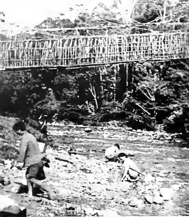
▲ THIS RATTAN SUSPENSION BRIDGE is typical of those built by the New Guinea natives. In the foreground are Dyak and Javanese servants of the expedition, washing cooking tins in the stream
