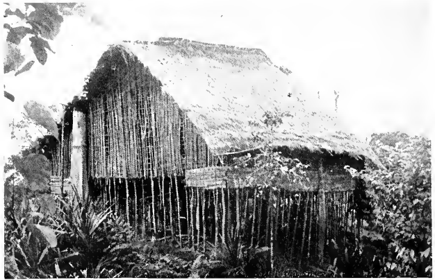
▲ MOST NEW GUINEA houses are built on supports like this one, which was found in a deserted garden on the upper Fly River
