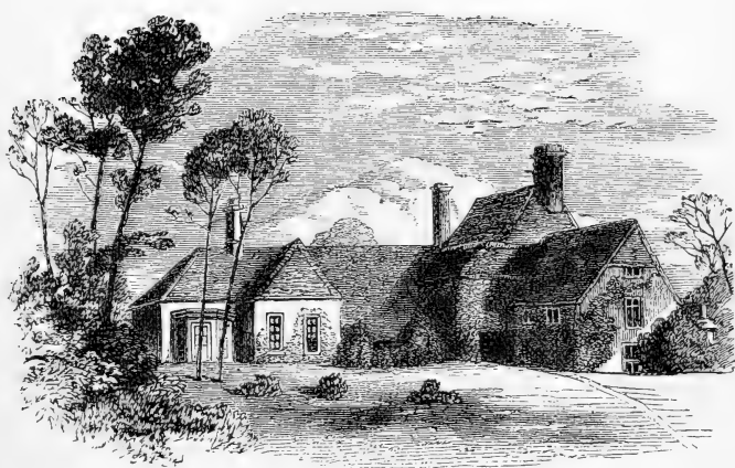
BACK VIEW OF WHITE'S HOUSE.
