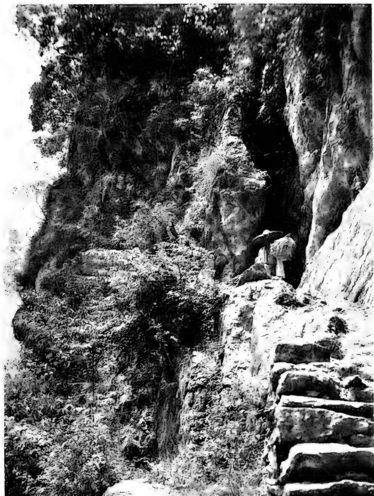
HIGHWAY LEAD THROUGH A NATURAL TUNNEL
