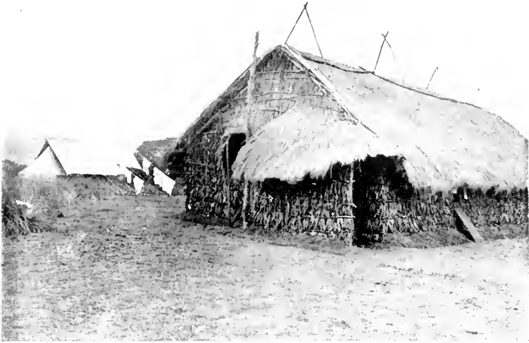
HOUSE ON BUGALLA, 1912-13. Barbed wire lightning conductor over supports on roof.
