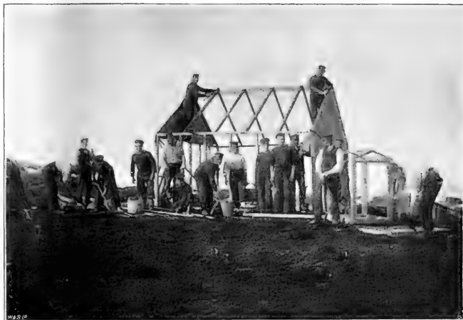
FIG. 2.—The erection of the Huts.
