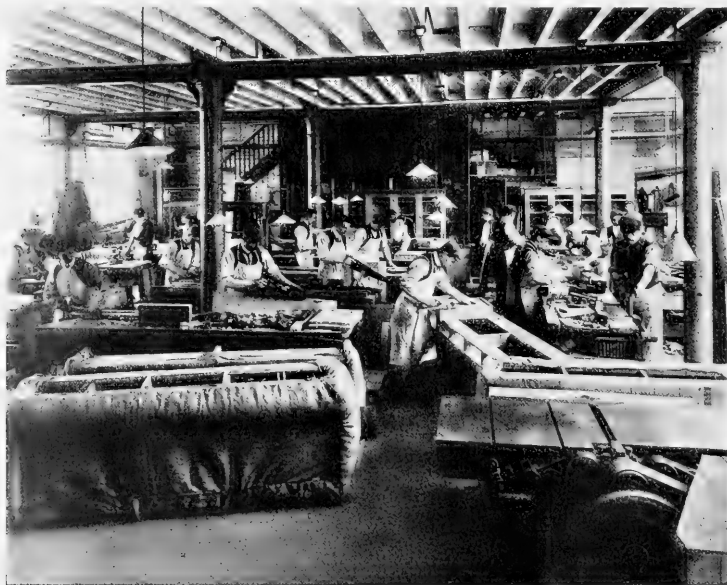
PART OF WOODWORKING SHOP FOR LABORATORY FURNITURE.
