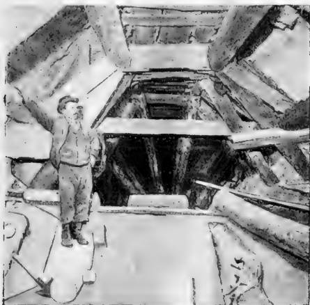
FIG. 3.—The timbering of the tunnel—six miles from the entrance.
