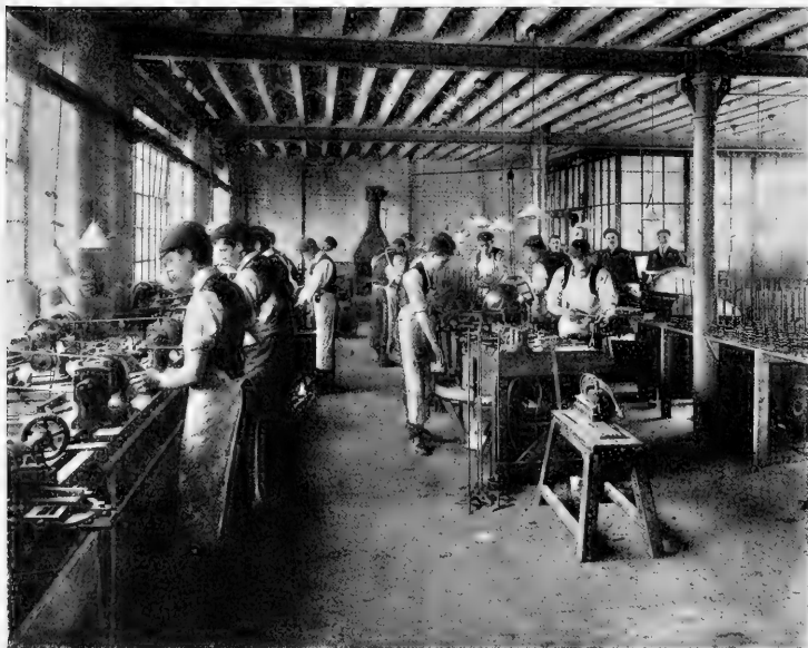
HEAVY METAL WORKING SHOP.
