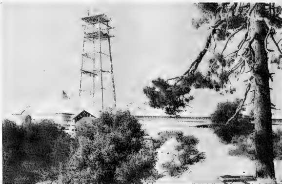
FIG. 2.—Vertical Celeostat or Tower Telescope, Mount Wilson Solar Observatory.
