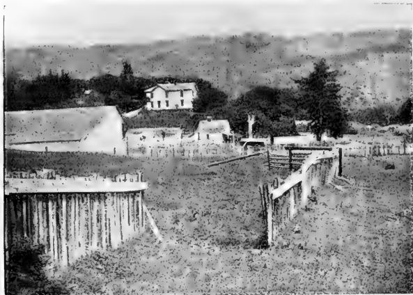
FIG. 1.—Fence parted by Earthquake Fault. The fault trace or fracture accompanying the earthquake is inconspicuous although the horizontal displacement is considerable. (Photograph by G. K. Gilbert.)
